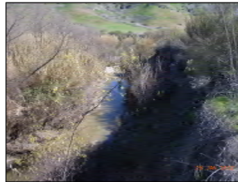
6 Upper Bank Geotechnical Instability
