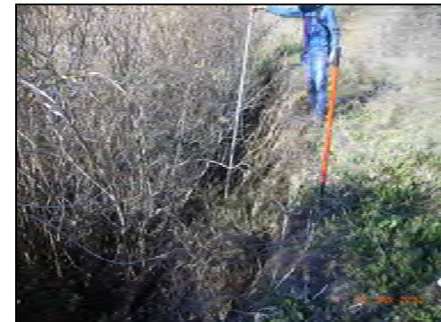
2 Upper Bank Geotechnical Instability
