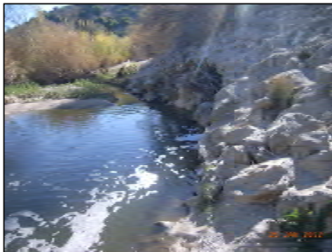
1 Undercut Grouted Riprap
