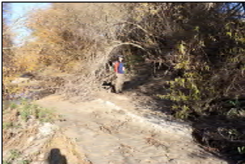
11 Stable Bank (looking u/s) Stability promoted by 6-foot high, vegetated, depositional berm along toe of bank. Floodplain connected, stable bank angle.
