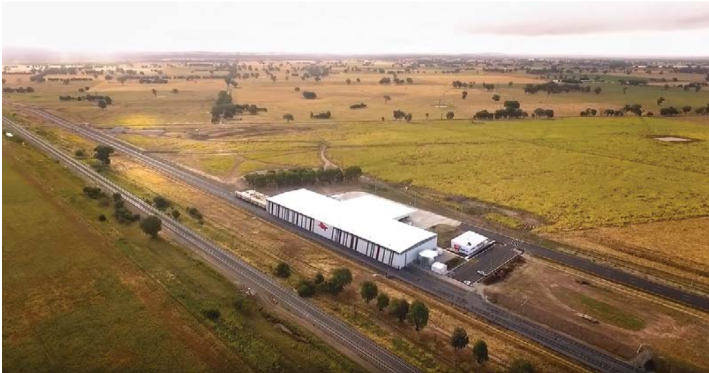
Figure 55 External view of Barnawartha intermodal terminal
