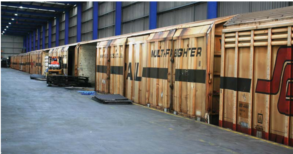
Figure 56 Internal view of Barnawartha intermodal terminal
