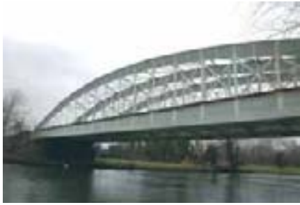
The triple 'bow and string' construction bridge carrying the branch line from Slough to Windsor.
