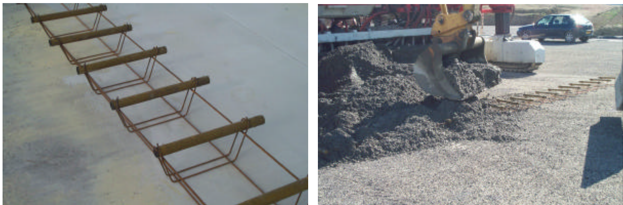
Figure I-7 : Dowels on basket / Concreting.
