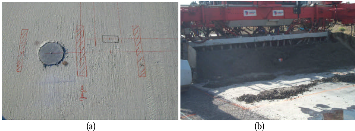
Figure II-8 : (a) place of the sensors / (b) concrete casting.
