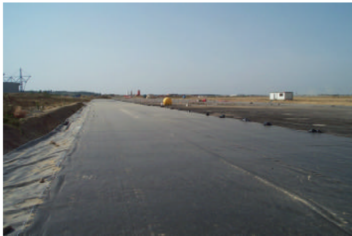
Figure I-14 : View of the geomembrane (extended over HUGA).
