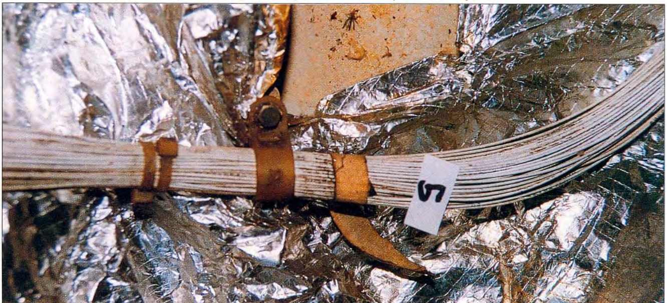
The tape wrap has slipped out of this clamp allowing the harness to spread and deform.
