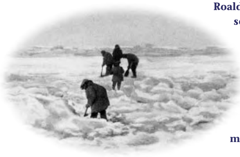
Levelling the ice field to prepare a "runway"
