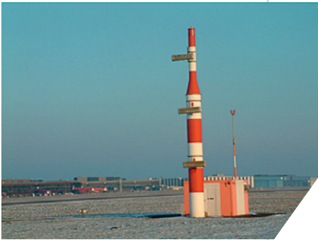
Localizer and Glide Path antennas
