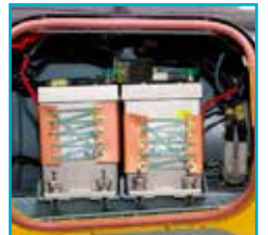
Second Battery Installation
