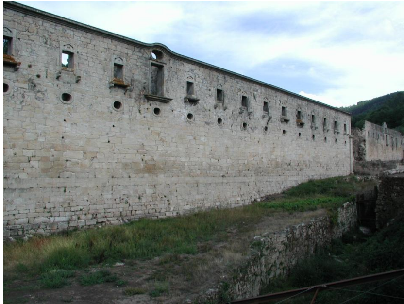
Fig.2 – Monastery of S. João de Tarouca, dormitory. (author's photography)
