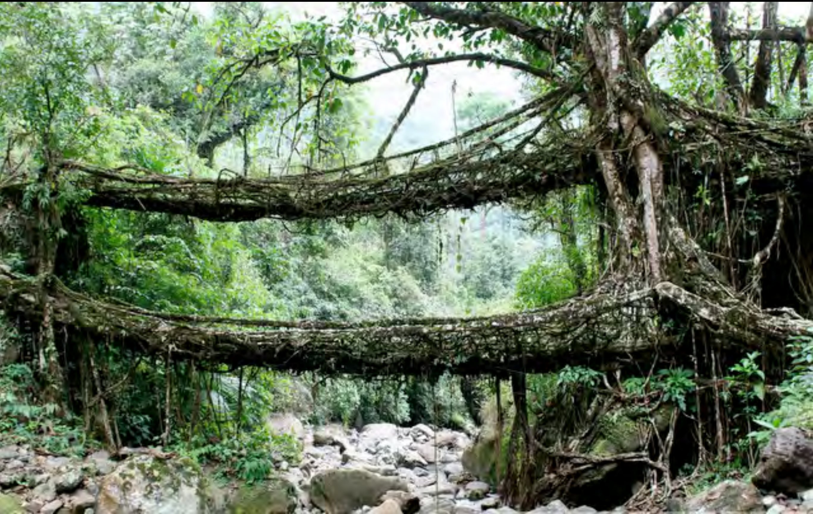
The living bridges of Cherrapunji, India are made from the roots of the Ficus elastica tree. ( http://rootbridges.blogspot.com/ )
