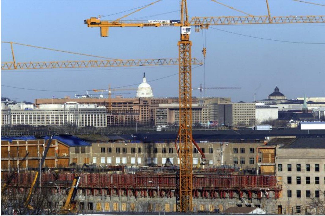
Phoenix Project Building Renovations Following The 9-11 Terrorist Attacks American Airlines Flight 77
