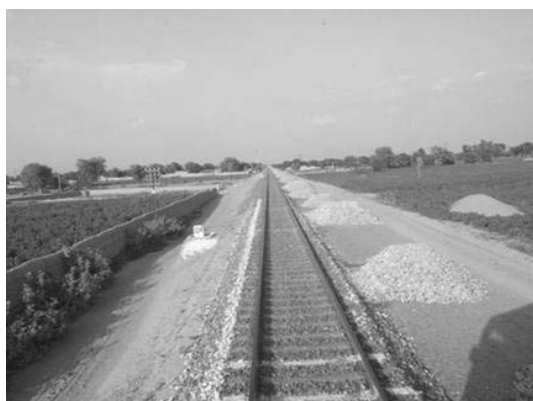
Photo: Double tracking work between Multan and Khanewal
