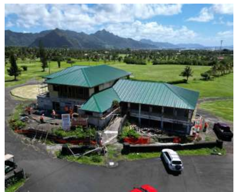
Country Club Renovation
