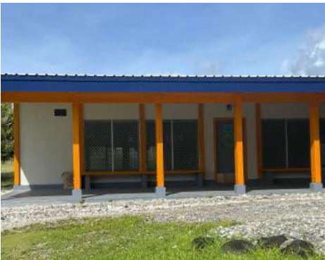
Ta'u ECE School Building
