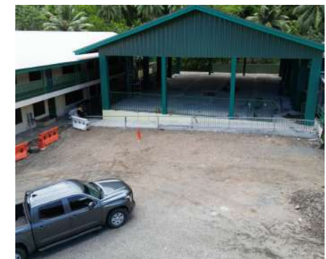
Tautalatasi Tuatoo ES New Multipurpose Building
