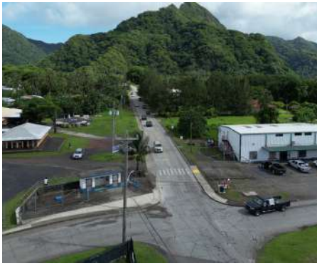
Road 018 New Road Construction Fagaima
