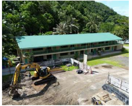
Afonotele ES Two-Story Classroom (Kitchen/Cafeteria)
