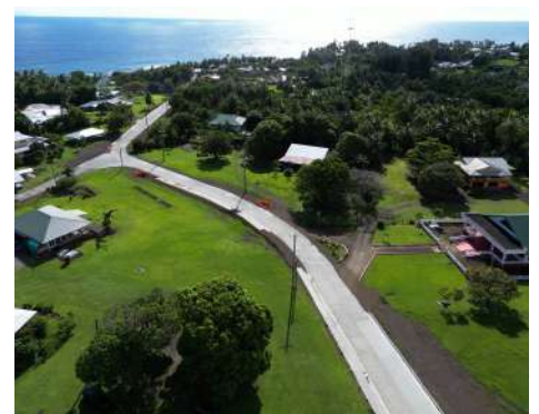
Route 003 Road Reconstruction Taputimu
