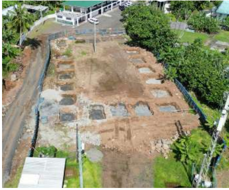
Alataua II ES Multipurpose Building
