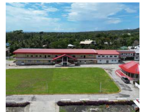
Peteli Academy Renovation & Repair
