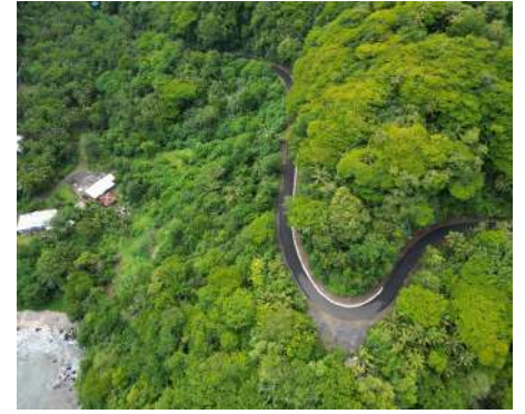
Amanave to Fagali'i Access Road
