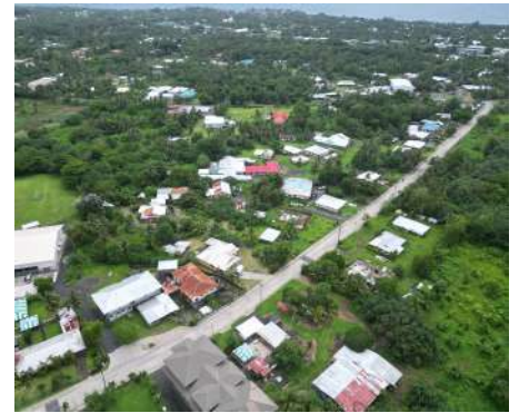
Route 13 Road Construction Malaeloa
