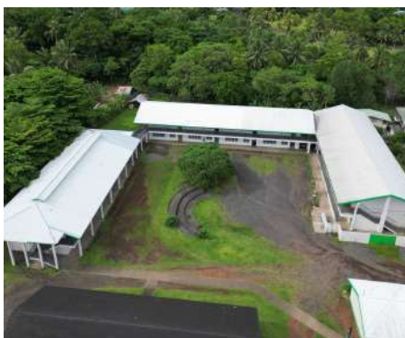
Lupelele ES Improved Classroom/Kitchen & Cafeteria
