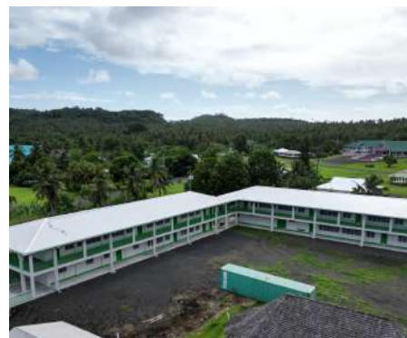
Lupelele ES Classrooms & Restrooms
