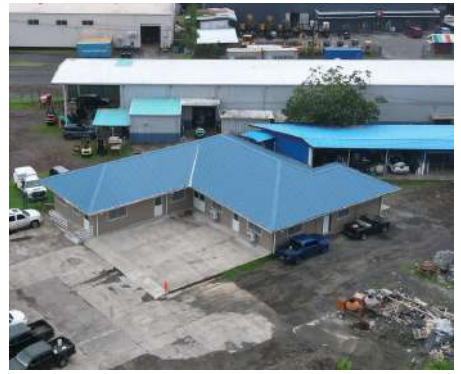
Parks & Recreational Office Renovation
