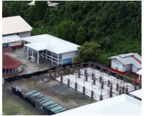
Fagaitua High School Classroom Improvements
