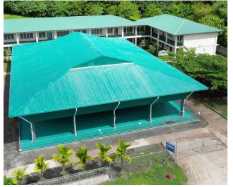
Fagali'i ES Multipurpose Building
