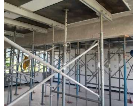
Tafuna HS Retrofitting Building
