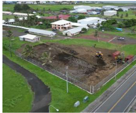
Tafuna HS JROTC Building
