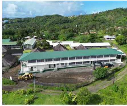
Pava'iai ES #2 Improved Kitchen, Cafeteria, & Classrooms
