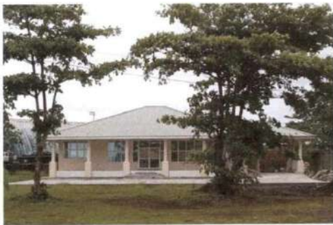
New Treasury Storage Bldg.
