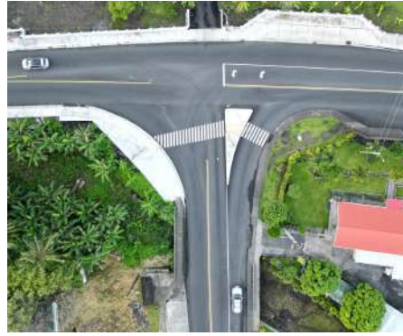
Island- Wide Safety Improvement Pavement Marking
