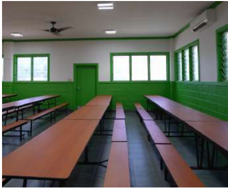
Lau'i ES Kitchen/Dining Improvements
