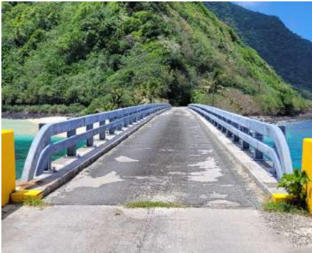
Ofu/Olosega Bridge Safety Rails
