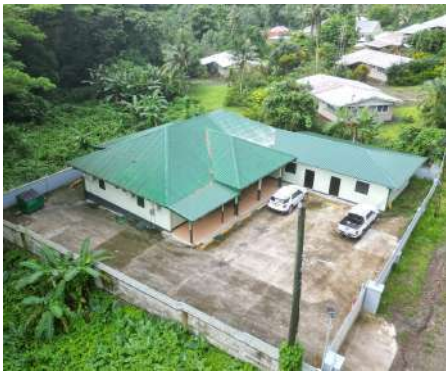
DHSS Malaeimi Shelter Renovation
