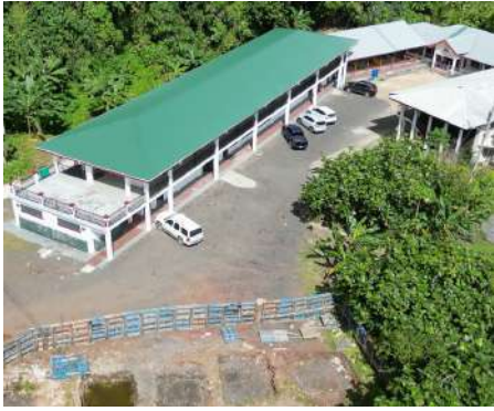
Alataua II ES Two-Story Building
