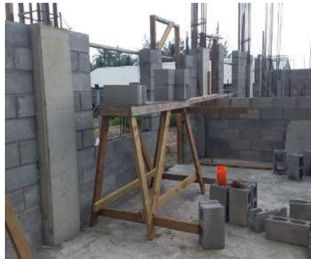
Olosega ES (Two Story Building)
