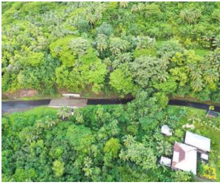
Poloa to Fagamalo Road Resurface
