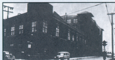
Sackett & Williams Printing Plant
