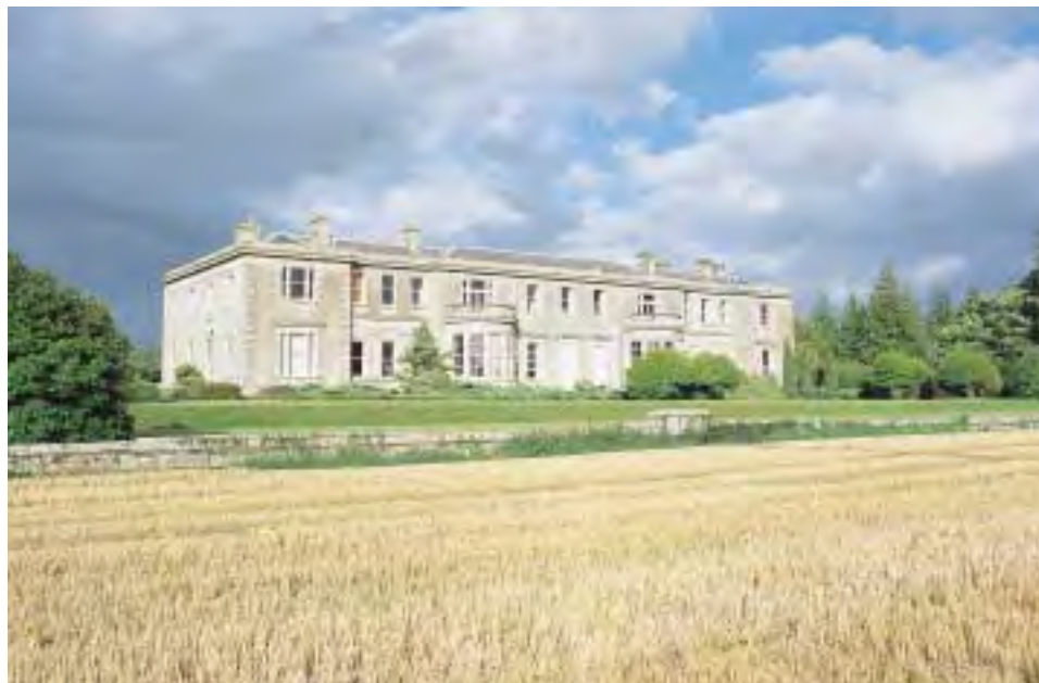
(fig. 41) OAK PARK HOUSE, Oak Park Demesne (c. 1760 & c. 1832)
