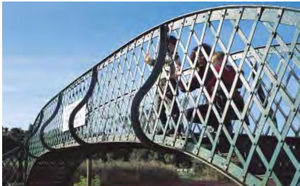
(fig. 72) FOOTBRIDGE, Muine Bheag railway station (c. 1880)
