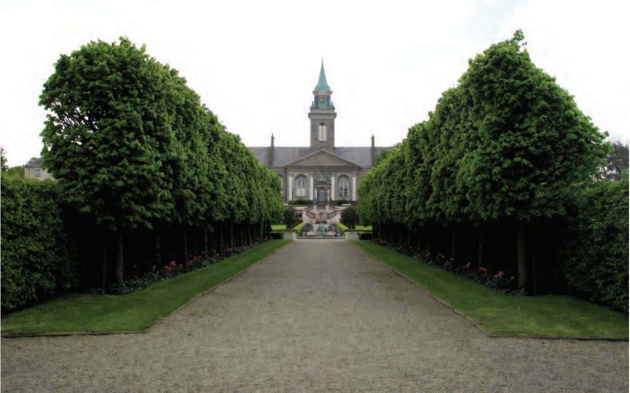
(fig. 15) ROYAL HOSPITAL (1680-4; 1705) Military Road, Kilmainham
