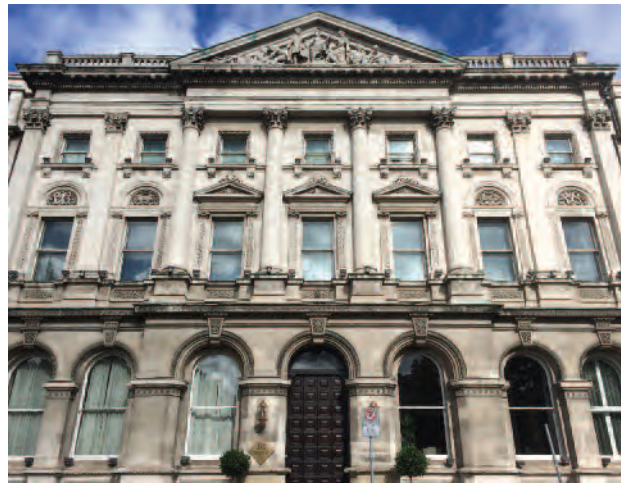
PROVINCIAL BANK OF IRELAND (1862-4) 1-2 College Street
