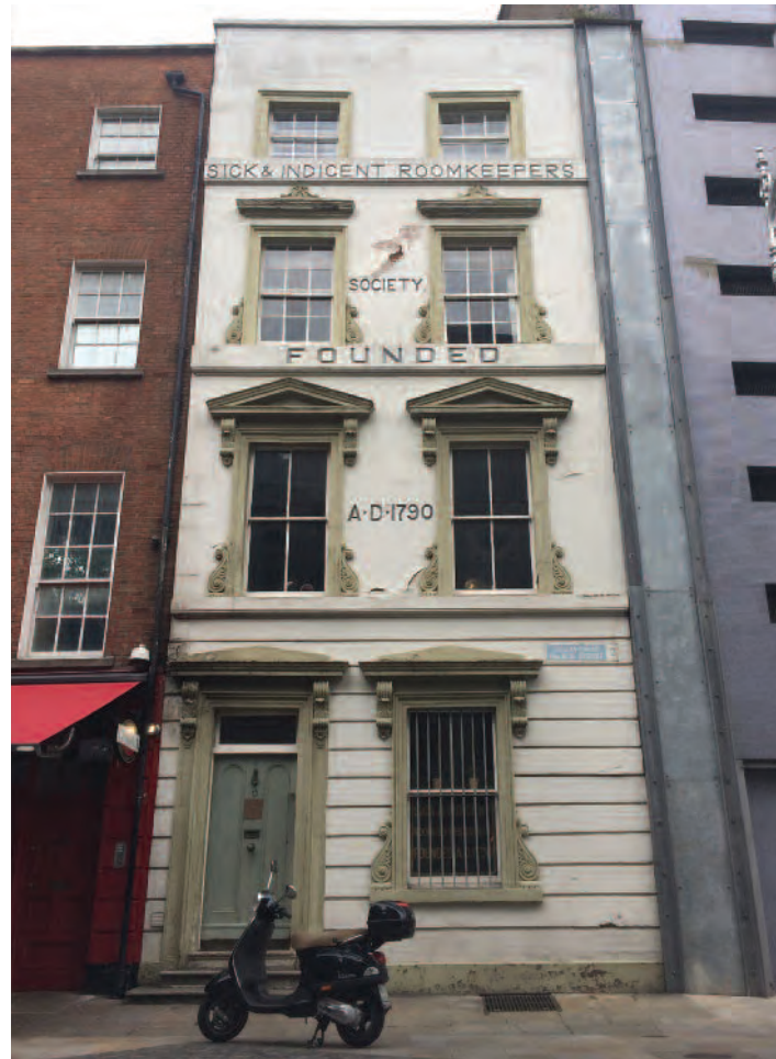
( fig. 50 ) SICK AND INDIGENT ROOMKEEPERS' SOCIETY 2 Palace Street
