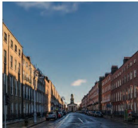
( fig. 76 ) ST STEPHEN'S CHURCH
