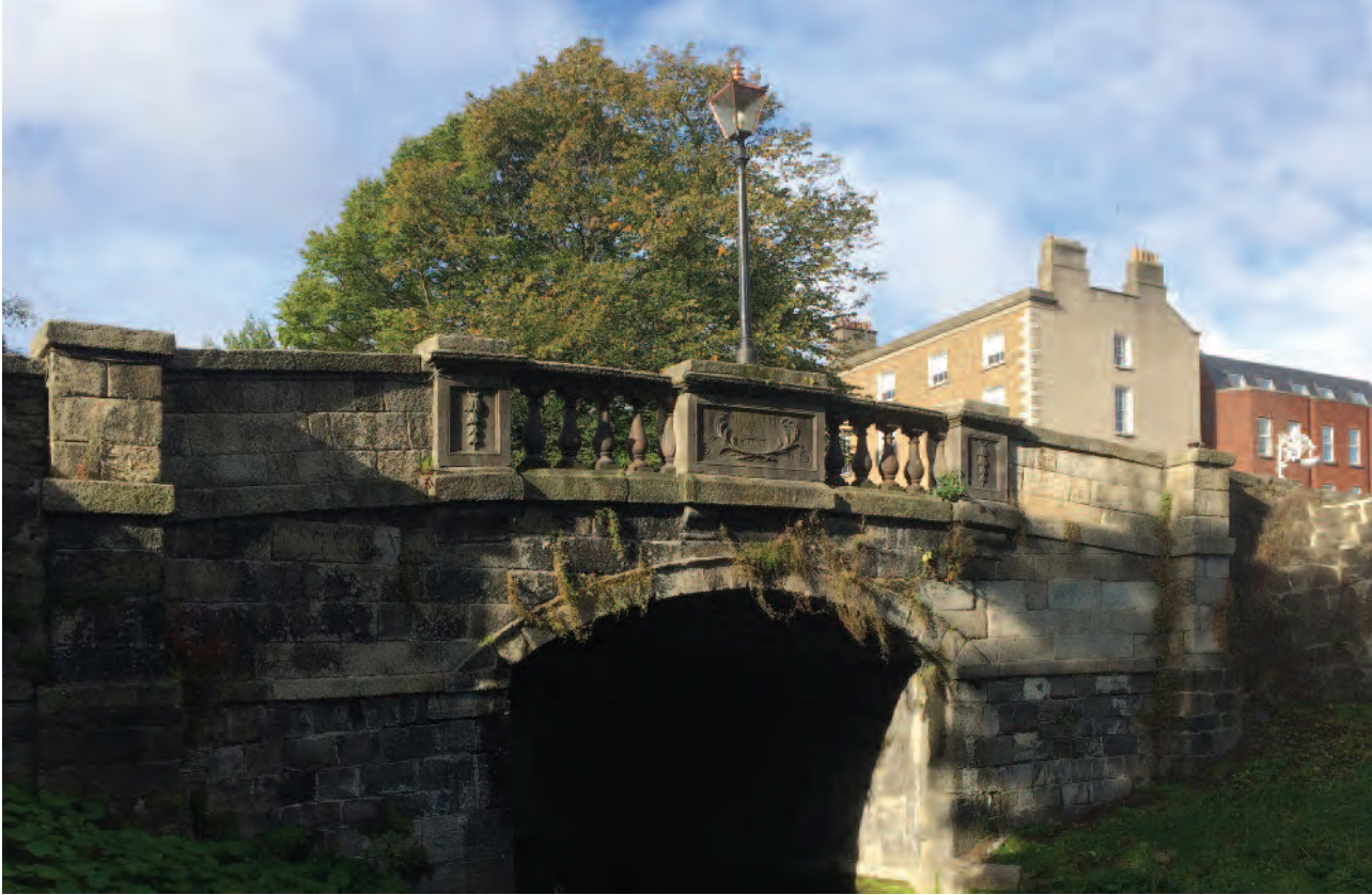
(fig. 54) HUBAND BRIDGE (1791)
