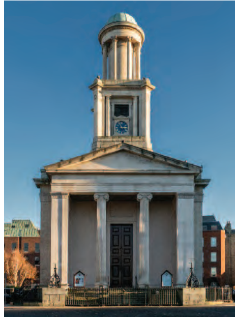
( fig. 75 ) ST STEPHEN'S CHURCH (1820-4; 1851) Mount Street Crescent
