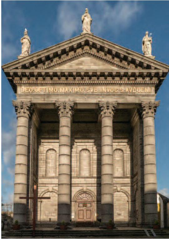
(fig. 73) ST AUDOEN'S CHURCH (1841-52; 1898-1902) High Street
