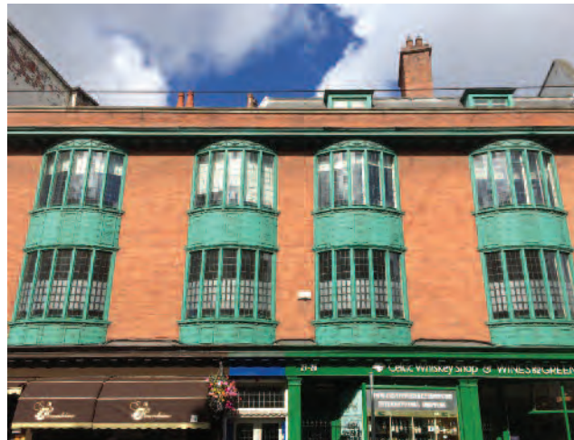
(fig. 134) MANSION HOUSE CHAMBERS (1910-1) 26-28 Dawson Street
