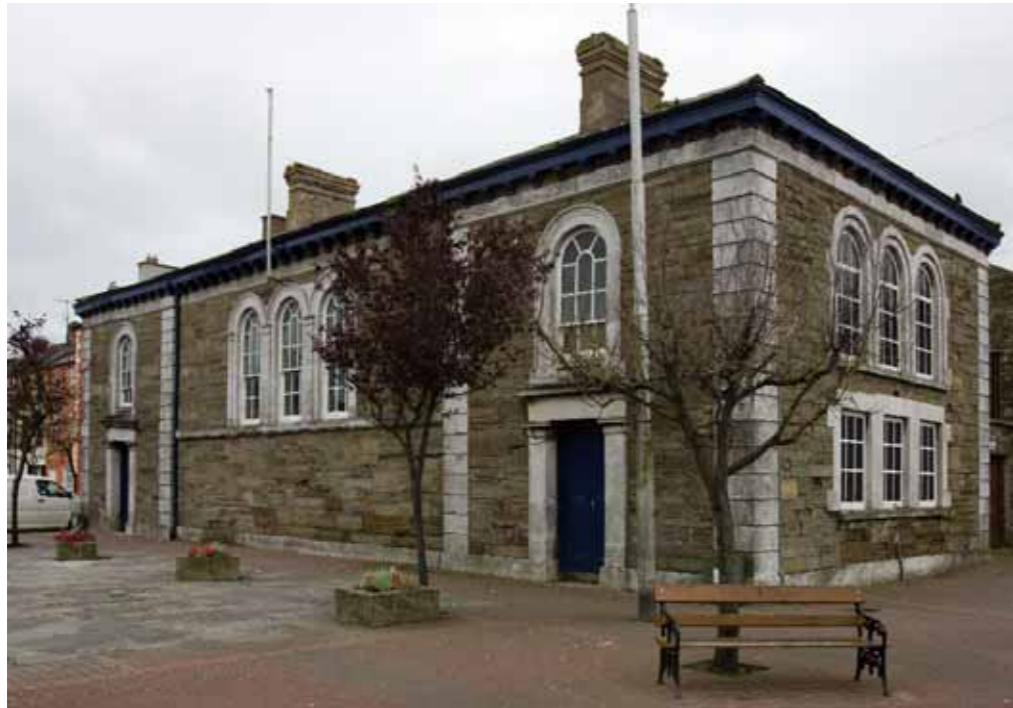
(fig. 107) YOUGHAL COURTHOUSE Market Square, Youghal (c.1845)
