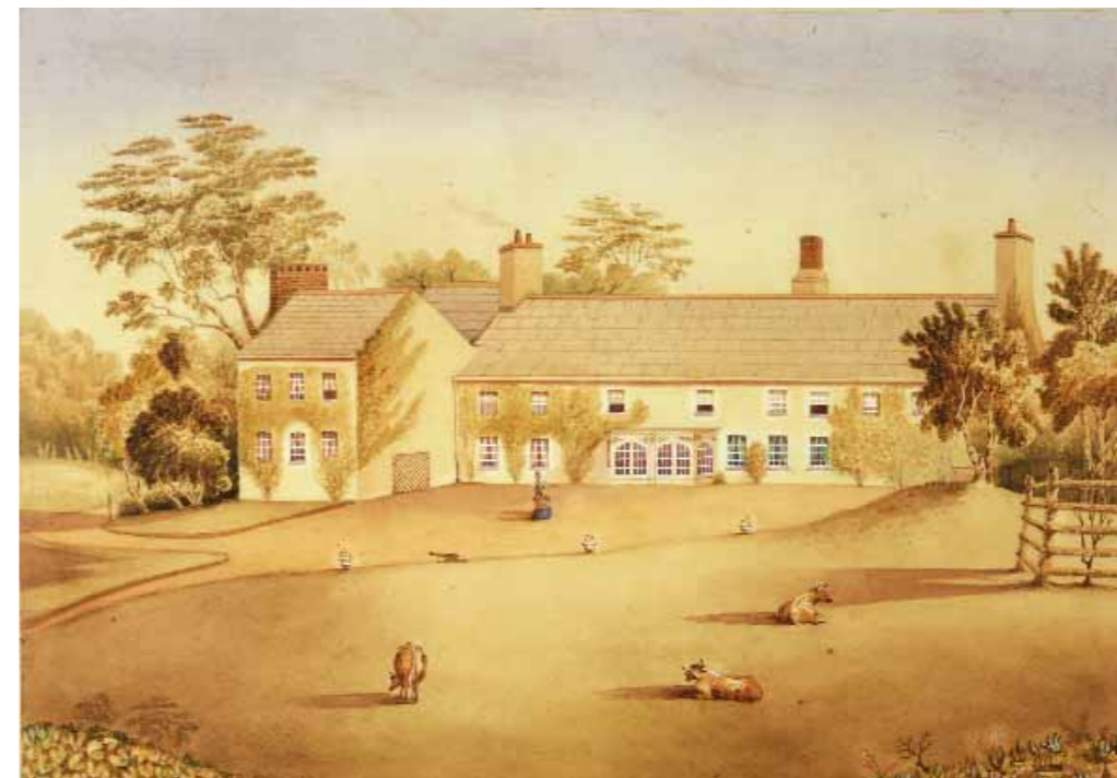
(fig. 52) AGHA DOE HOUSE Aghadoe Td. (c.1700)
