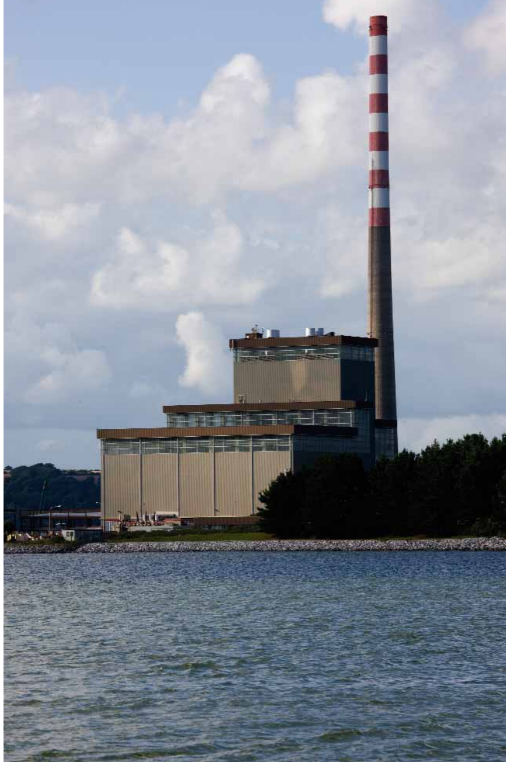
(fig. 198) AGHADA GENERATING STATION Ballincarroonig Td. (1978)
