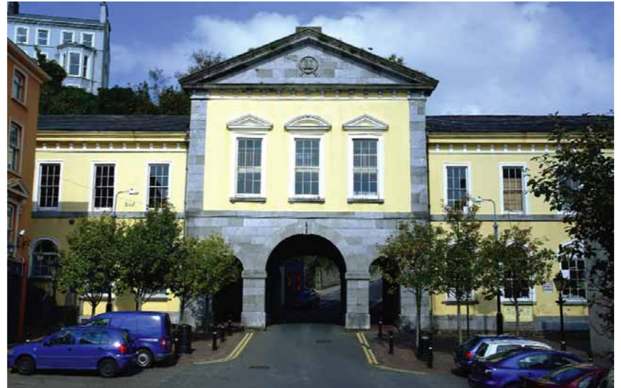
(fig. 126) FORMER TOWN HALL NOW COBH LIBRARY) Casement Square, Cobh (c.1840)
