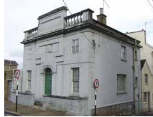
(fig. 95) FORMER BANK Emmet Place, Youghal (c.1810)
