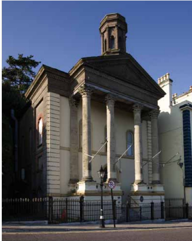
(fig. 145) FORMER METHODIST CHURCH (LATER THE PILLARS BAR) Westbourne Place, Cobh (1873)
