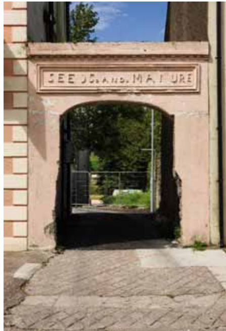
(fig. 97) CARRIAGE ARCH Rock Street, Cloyne (c.1840)
