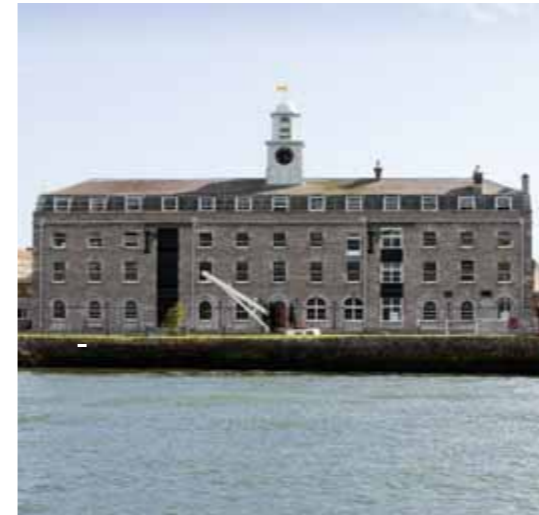
(fig. 72) FORMER NAVAL STORE (NOW NAVAL OFFICE) Haulbowline Island Td. (1822)
