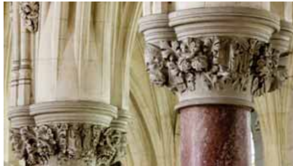
(fig. 129) INTERIOR DETAIL, ST COLMAN'S CATHEDRAL Cathedral Place, Cobh (1868-1919)
