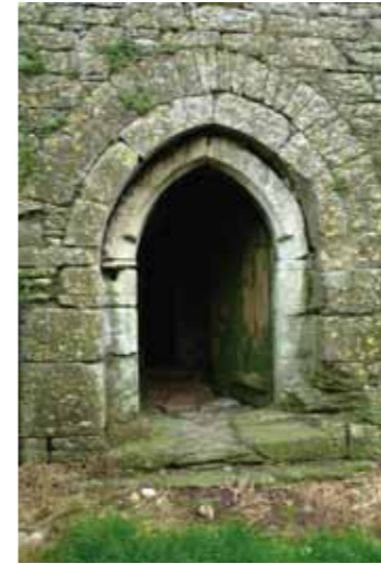
(fig. 20) DOORWAY, INCHICRENAGH CASTLE Castlerichard Td. (1592) Also called Castle Richard, the construction of the original stronghold on this site is attributed to Richard Fitzgerald, the first Seneschal of Imokilly (1422). The castle was repaired or rebuilt by Thomas 'Geannagh' Fitzgerald as evidenced by the cut-limestone surround of the pointed-arch door-opening which bears the date 1592 and initials T. G. in false relief.
