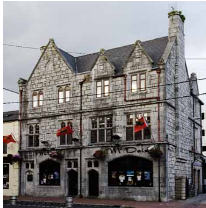
(fig. 111) FORMER SHOPS (NOW McDAID'S PUB) Main Street, Midleton (1851)
