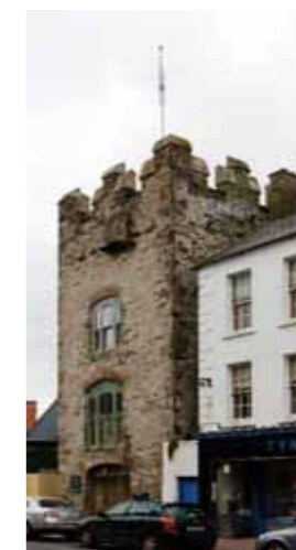
(fig. 17) TYNTE'S CASTLE North Main Street, Youghal (c.1450)
