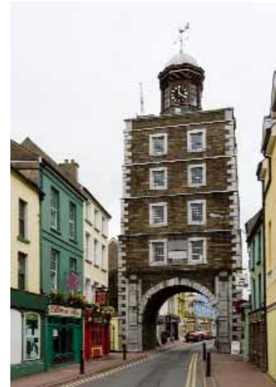
(fig. 34) THE CLOCK GATE South Main Street/ North Main Street, Youghal (1777)
