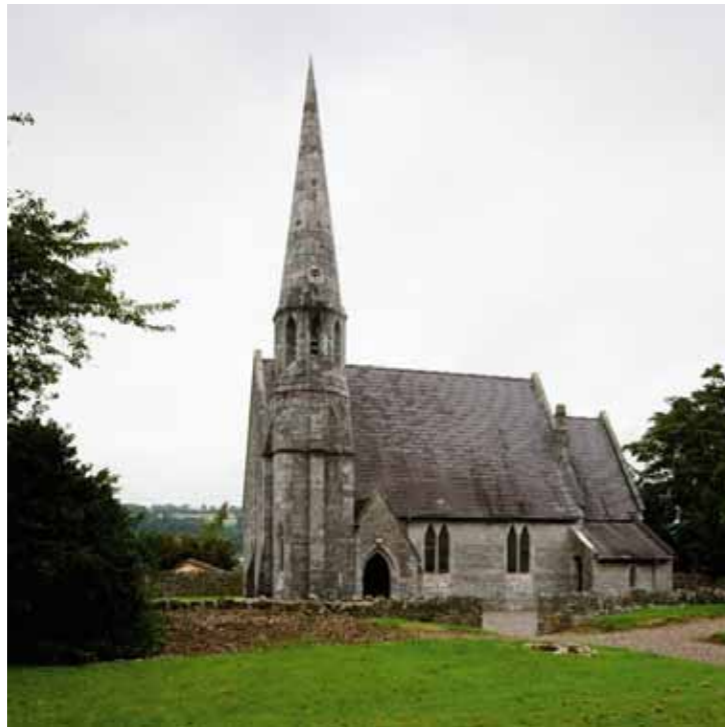
(fig. 140) ST LAPPAN'S CHURCH OF IRELAND CHURCH Little Island (1865)
