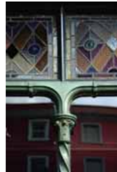
(fig. 125) METAL IMITATING TIMBER, THE MAURETANIA 14 Casement Square, Cobh (c.1855)
