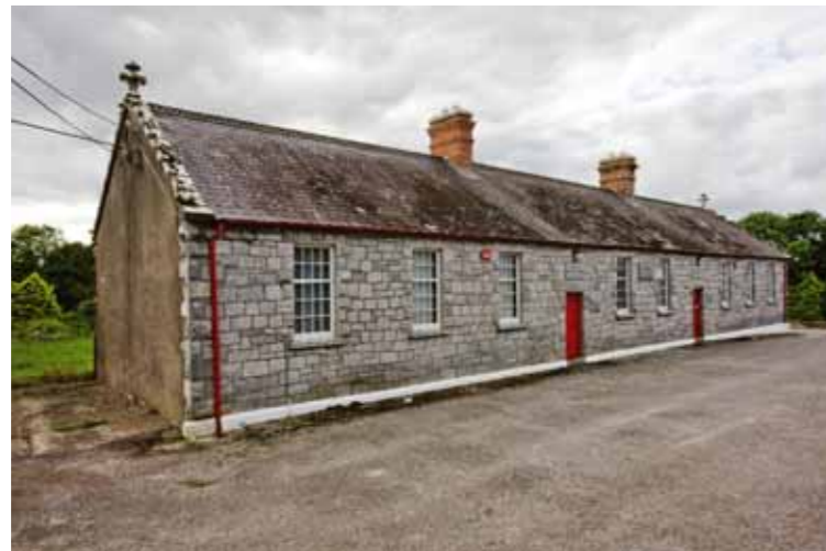
(fig. 149) FORMER NATIONAL SCHOOL (NOW CASTLEMARTYR ENTERPRISE CENTRE) Park Street, Castlemartyr (1889)
