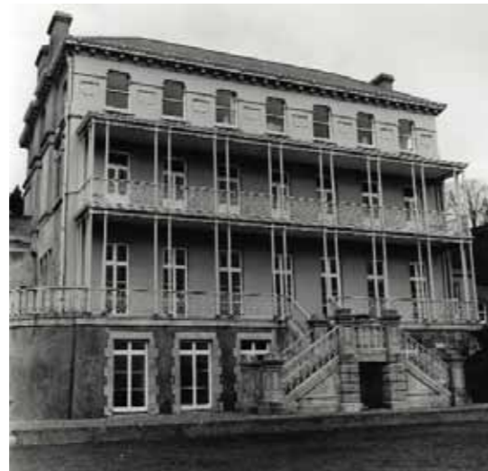
(fig. 117) FORMER ADMIRALTY HOUSE Beechmount Park, Cobh (1886)
