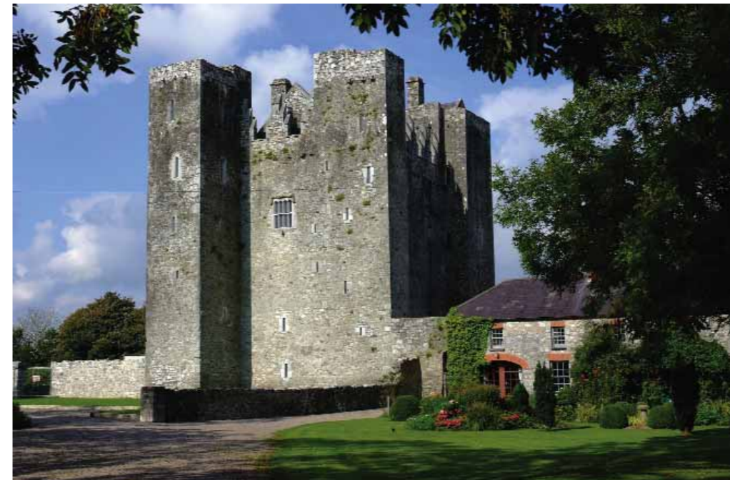
(fig. 21) BARRY'S COURT CASTLE Barryscourt Td. (c.1585) This was the main stronghold of the Barry family from the late twelfth century. The present appearance of the castle dates from c.1585, when it was extensively remodelled by David Barry. The original castle is attributed to William de Barri whose uncle, Gerald of Wales, is believed to have written his famous History and Topography of Ireland (1184) here.
