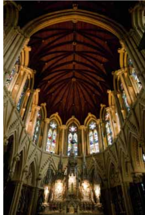
(fig. 128) THE CEILING, ST COLMAN'S CATHEDRAL Cathedral Place, Cobh (1868-1919)
