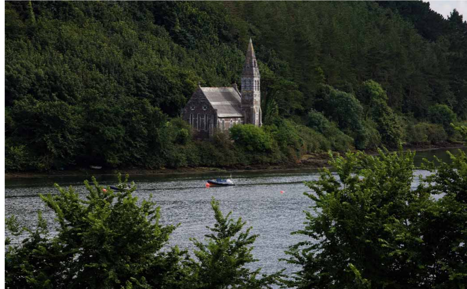
(fig. 141) HOLY TRINITY CHURCH OF IRELAND CHURCH IN ITS SETTING Garranekinnefeake Td. (1865)
