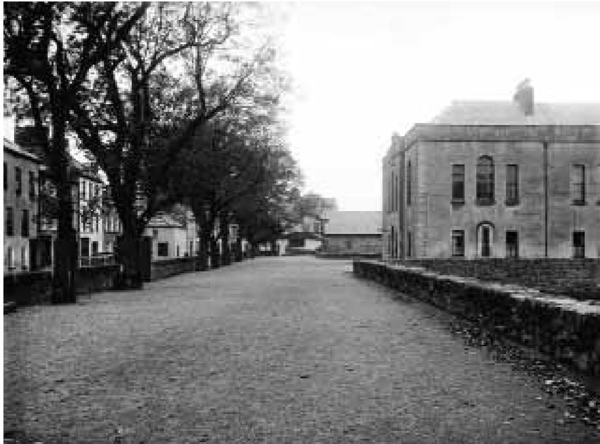
(fig. 33) TOWN HALL The Mall, Youghal (1779)
