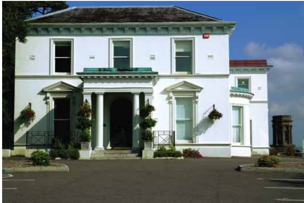
(fig. 158) FORMER CARRIG HOUSE (NOW COBH UDC OFFICES) Spy Hill, Cobh (c.1860)
