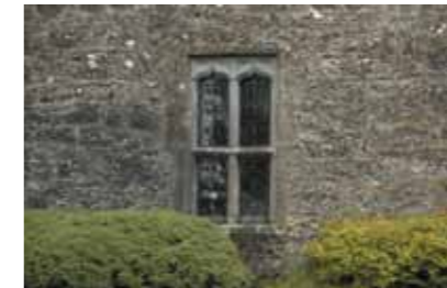
Double-light window of about 1550, in the ground floor of the towerhouse.
