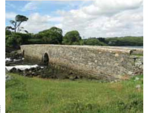
(fig. 74) ARDBEAR BRIDGE Ardbear (c.1820)
