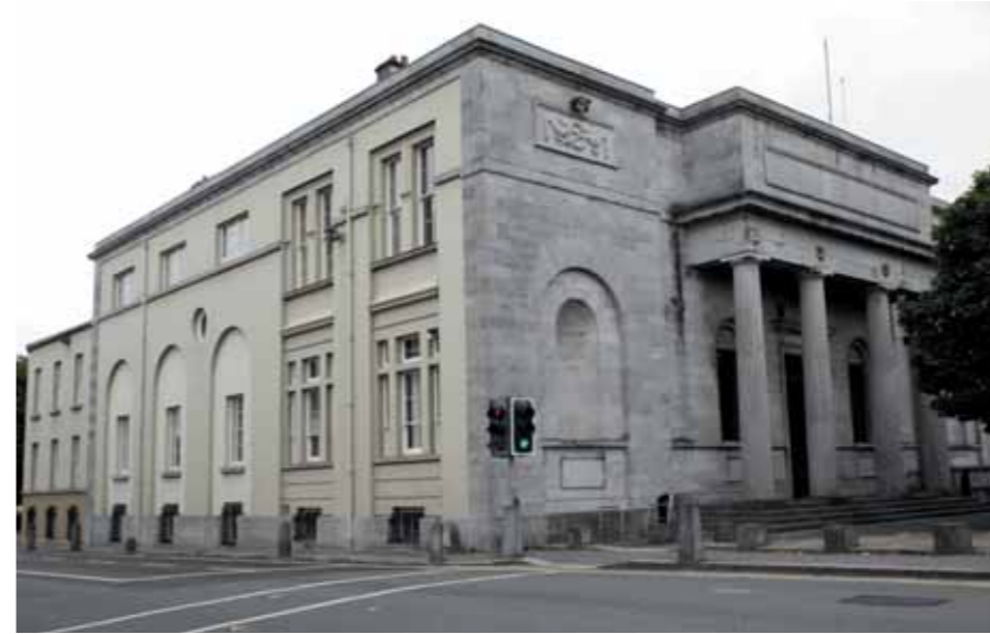
(fig. 82) GALWAY COURTHOUSE Courthouse Square Galway (1812-15)
