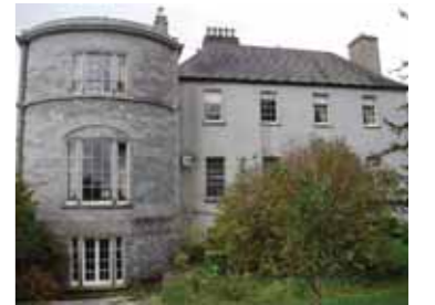
Side elevation, showing the older block to the rear.
