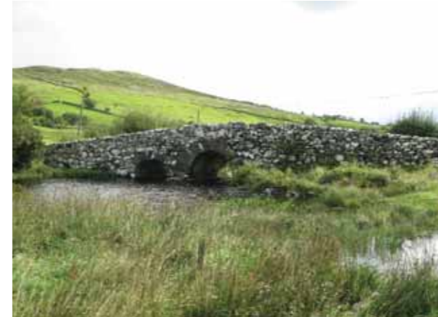
(fig. 16) THE QUIET MAN BRIDGE Leam East /Derryerglinna (c.1800)
