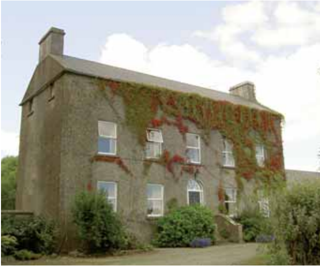
RICHMOUNT HILL Screeboge, near Carrickboy (c. 1720)
