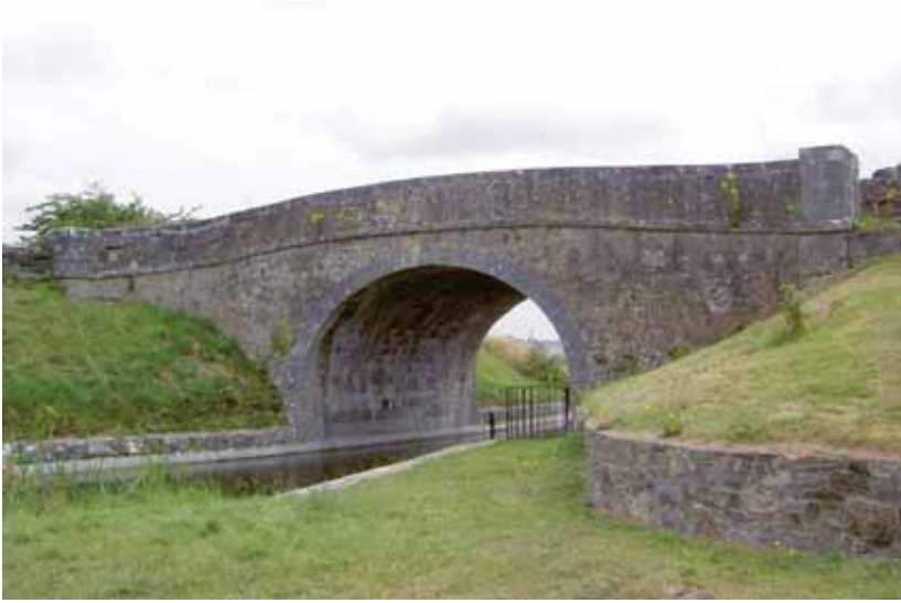
TOOME BRIDGE Toome (Shrulle Barony) (c. 1815)
