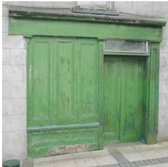
( fig. 84 ) MAIN STREET GRANARD (c. 1820; shopfront c. 1880)
