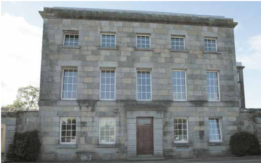
(fig. 48) LONGFORD PRISON Battery Road, Longford Town (c. 1825)
