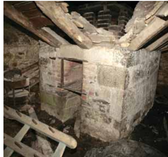
GRILLAGH MILL Grillagh, near Killashee (c. 1800, extended c. 1860)
