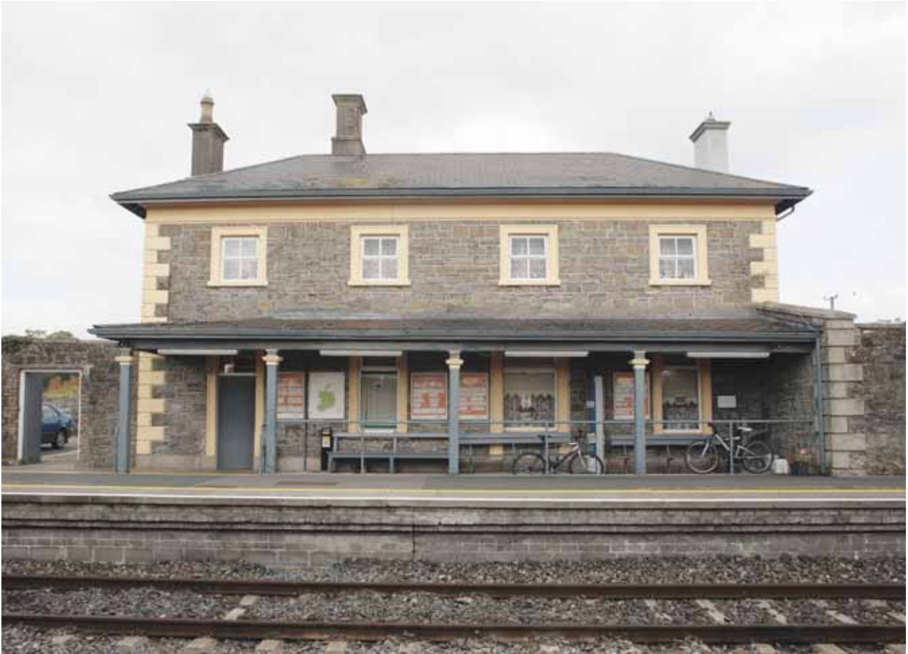
(fig. 51) EDGEWORTHSTOWN STATION Edgeworthstown (1855)
