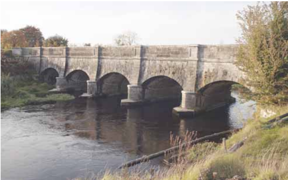
( fig. 50 ) WHITWORTH AQUEDUCT Drumanure/Cloonbrin (1814-7)
