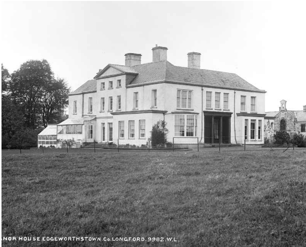
(fig. 31) EDGEWORTHSTOWN HOUSE Edgeworthstown (c. 1725; altered between c. 1782-1812 and c. 1870)
