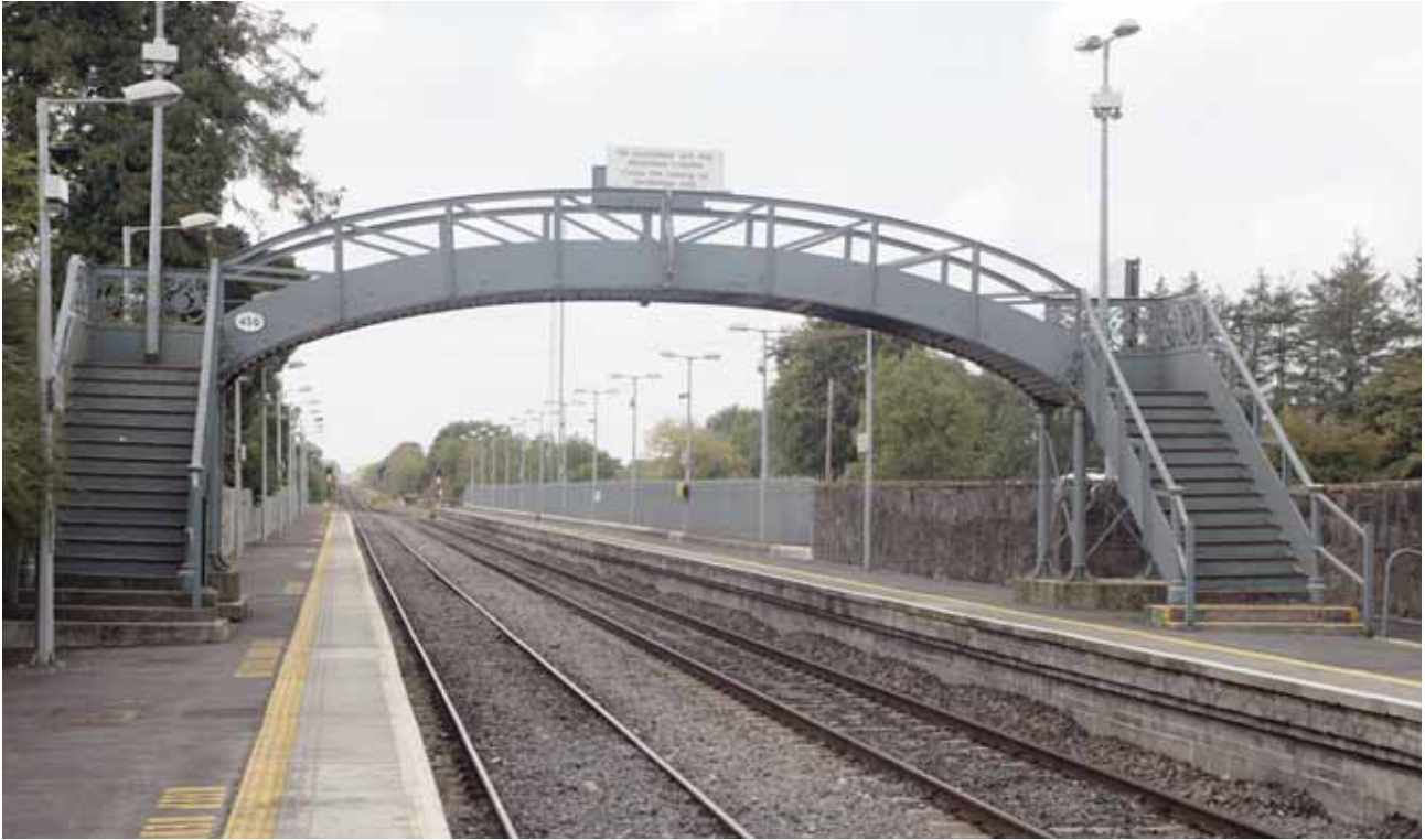
(fig. 52) EDGEWORTHSTOWN STATION Edgeworthstown (1855 or c. 1885)
