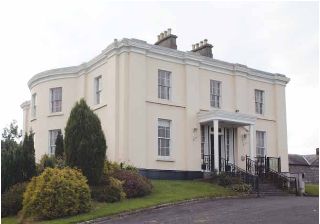
(fig. 72) COOLAMBER MANOR Cloonshannagh or Coolamber Manor Demesne (c. 1830)
