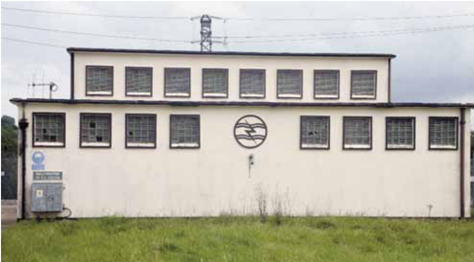
( fig. 92 ) BALLYMAHON ESB SUBSTATION Cornacarta (c. 1950)
