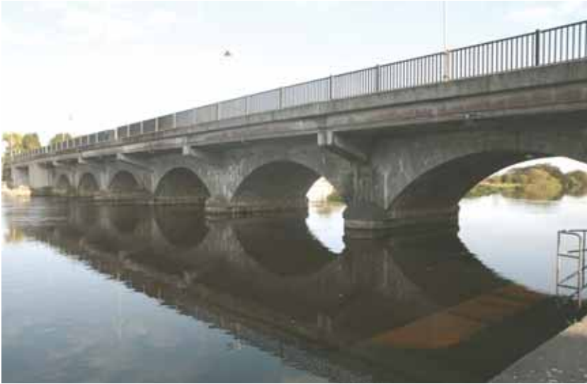
LANESBOROUGH BRIDGE Lanesborough (c. 1835-43; altered 1993)
