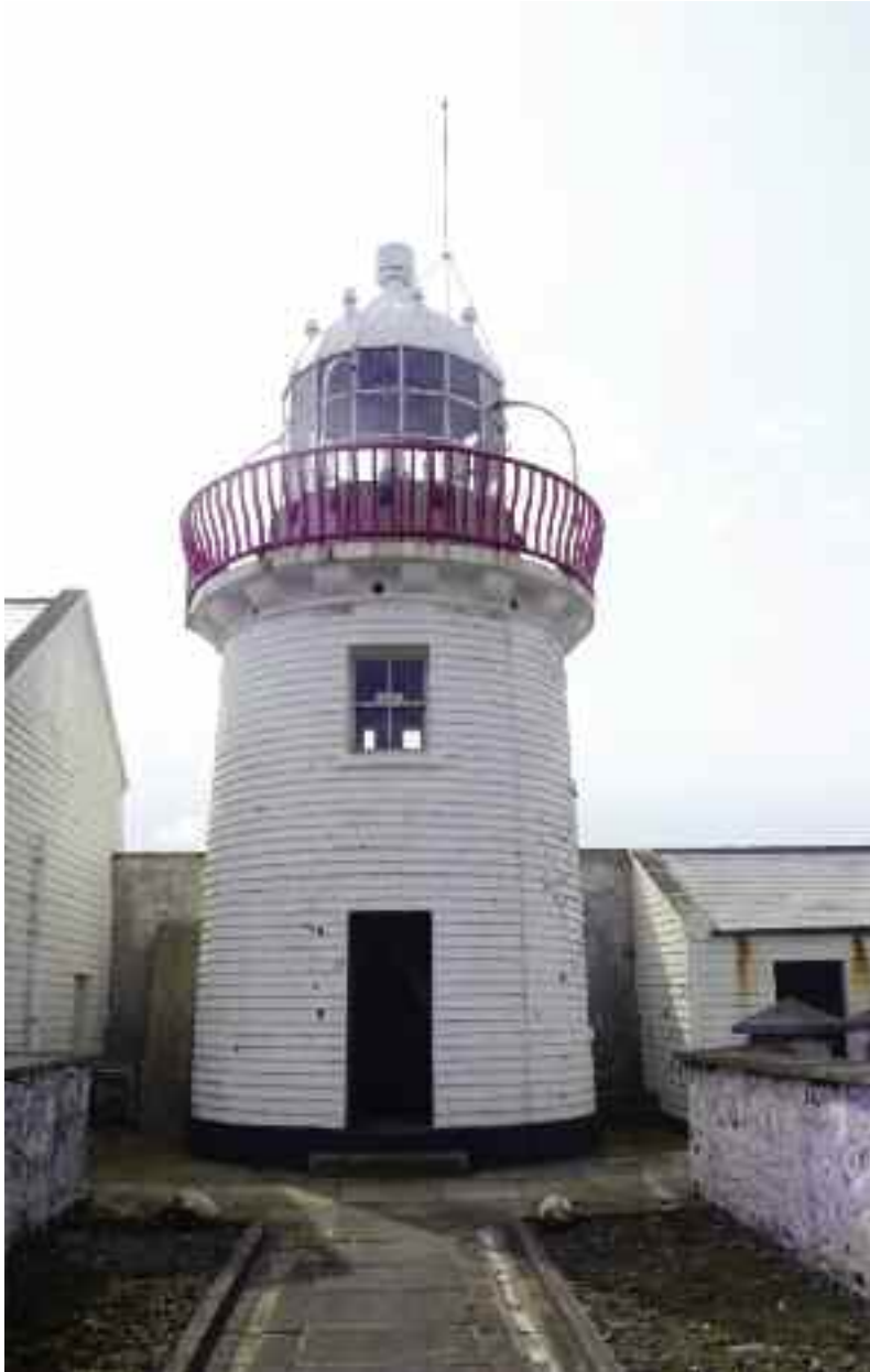
(fig. 37) INISHGORT LIGHTHOUSE Inishgort Island (1827-8)
