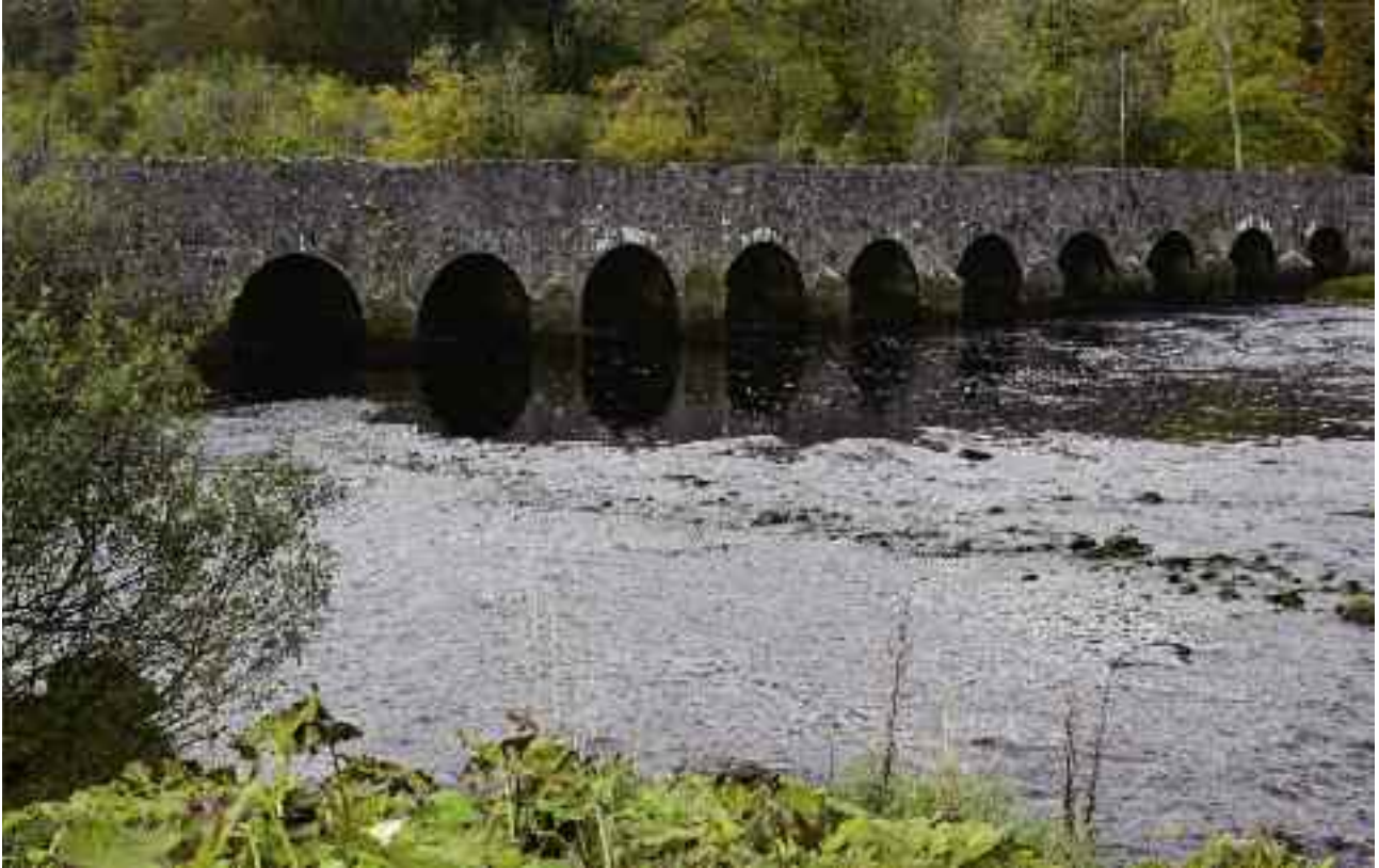
PALMERSTOWN BRIDGE Doonamona/Castlereagh
