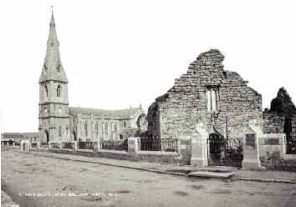
(fig. 64) SAINT MUREDACH'S CATHOLIC CATHEDRAL Cathedral Road, Ballina (1827-37)
