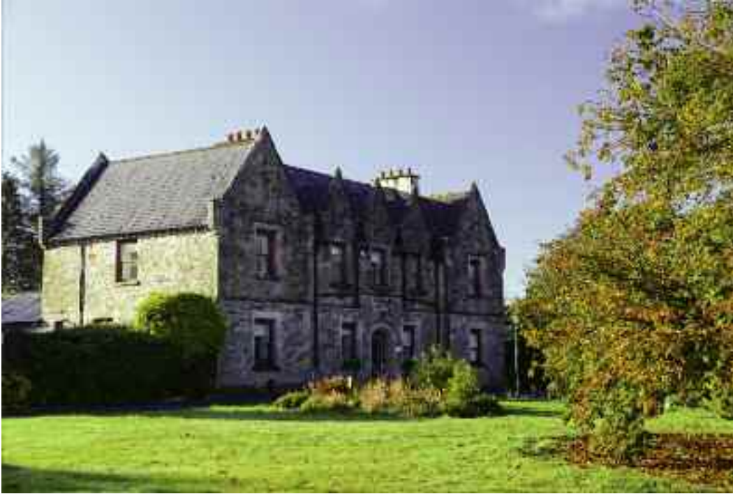
(fig. 80) SWINFORD UNION WORKHOUSE Bridge Street, Swinford (1840-2)
