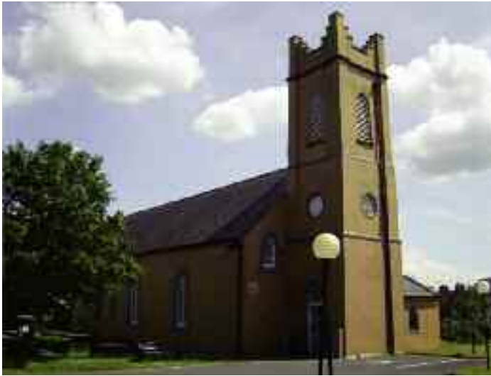
(fig. 139) SAINT MARY'S CHURCH (Ballinrobe) Church Lane, Ballinrobe (1815-8)
