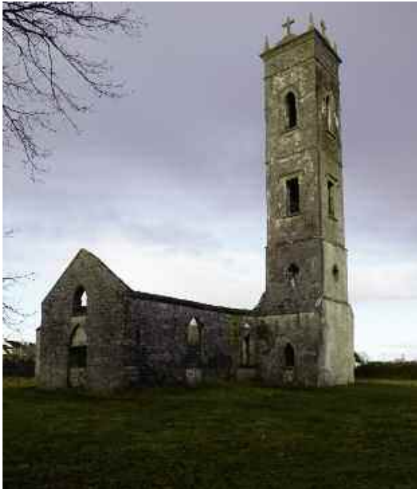
(fig. 63) BALLINROBE CATHOLIC CHAPEL Castlebar Road, Ballinrobe (1815-9)
