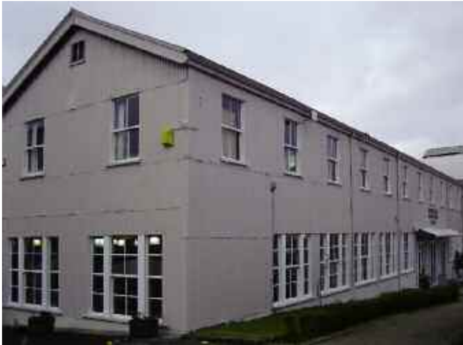
(fig. 121) FOXFORD WOOLLEN MILLS Lower Main Street, Foxford (established 1892)
