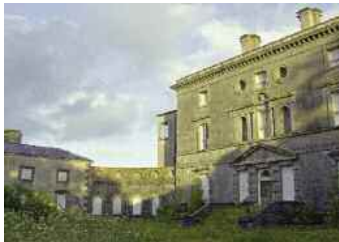
(fig. 18) HAZELWOOD HOUSE Hazelwood Demesne
