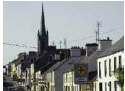
(fig. 123) EMLAGHFAD PARISH CHURCH Lord Edward Street, Ballymote
