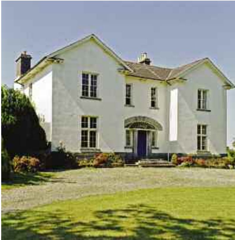
(fig. 11) CASTLETOWN HOUSE Cottlestown (c. 1820)
