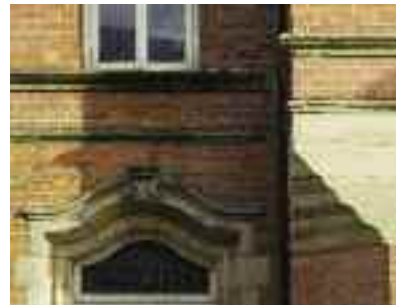
(fig. 173) YEATS MEMORIAL BUILDING Lower Knox Street, Sligo
