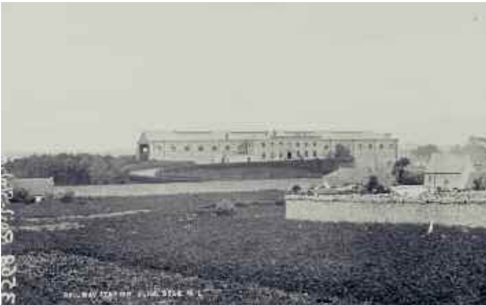
(fig. 46) MACDIARMADA (SLIGO) RAILWAY STATION Knappagh Road (c.1860)
