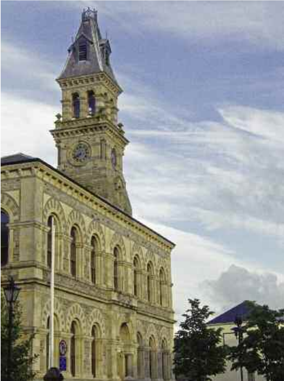
(fig. 68) SLIGO TOWNHALL Quay Street, Sligo (c.1865)
