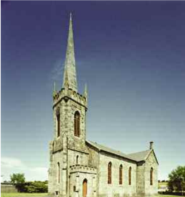
(fig. 122) EMLAGHFAD PARISH CHURCH Lord Edward Street, Ballymote (1818)
