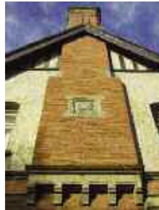
(fig. 172) YEATS MEMORIAL BUILDING Lower Knox Street, Sligo
