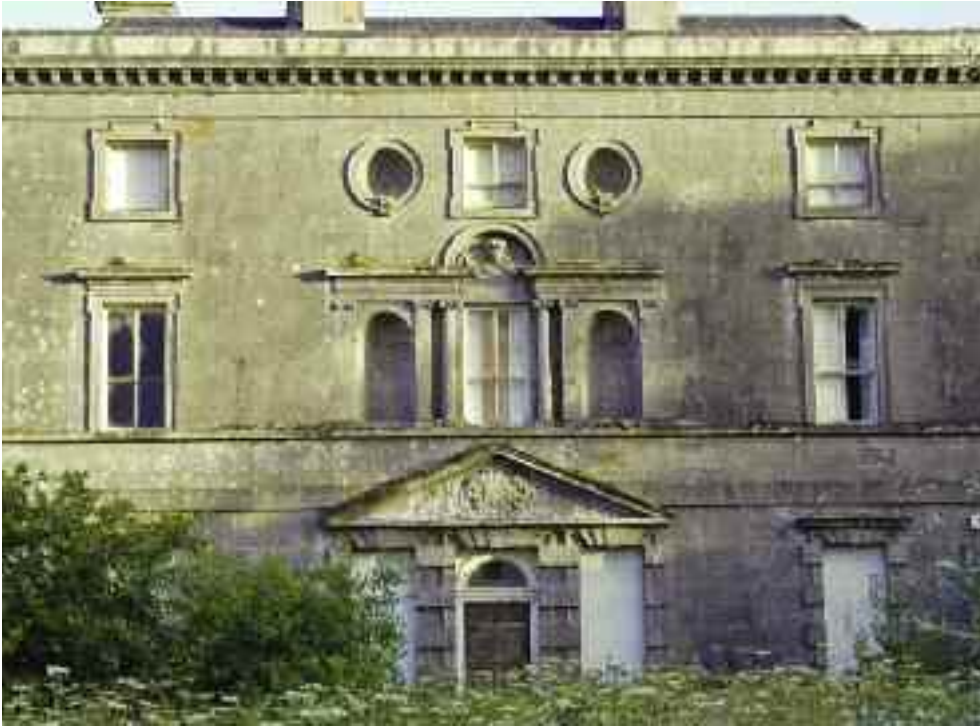
(fig. 17) HAZELWOOD HOUSE Hazelwood Demesne
