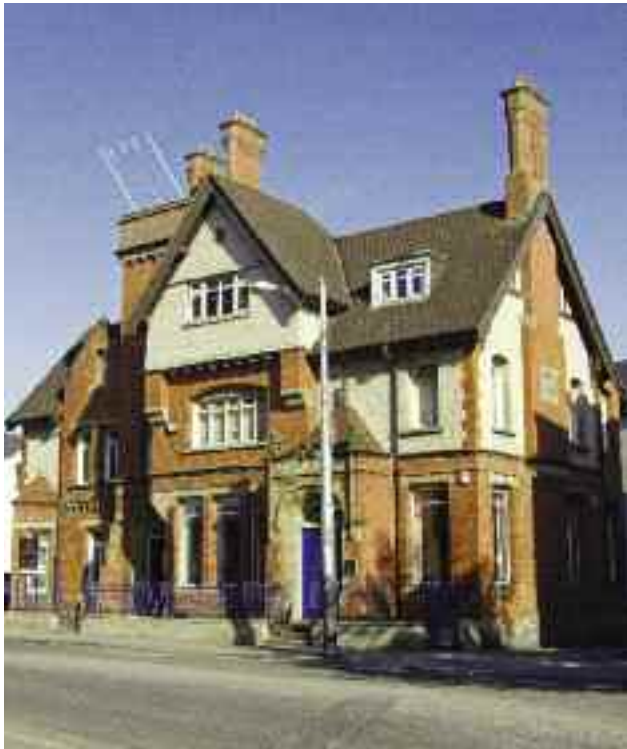
(fig. 171) YEATS MEMORIAL BUILDING Lower Knox Street, Sligo (c.1899)
