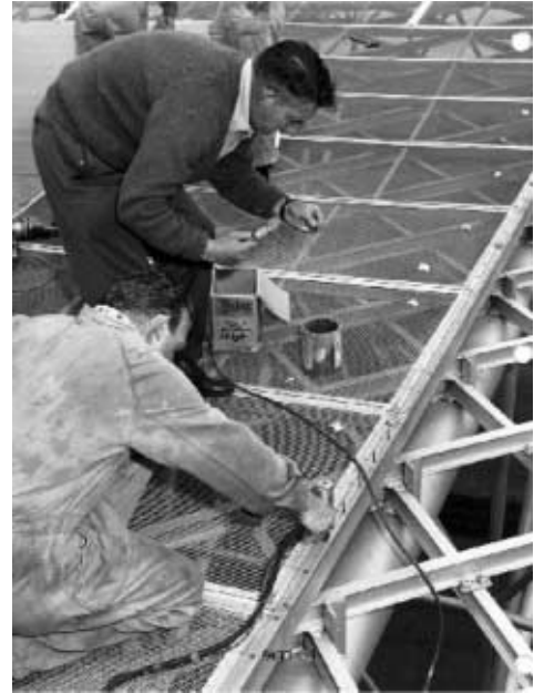
Figure 17 John Bolton and Fox Mason resurfacing the dish in 1973 (Photo: CSIRO).
