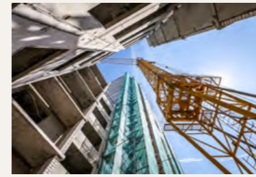
Galleries Shopping Centre in Wigan:
