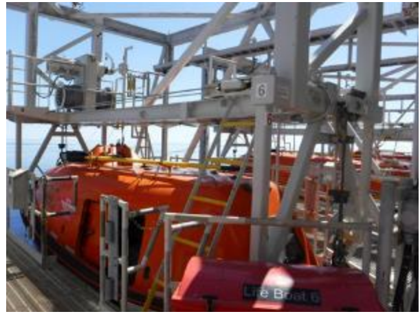
Figure 7: Lifeboat Station No. 6 davit. Figure depicts raised landing where winch is located. Credit: Palfinger, dated May 2015.
