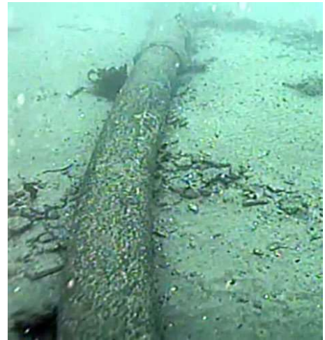
Figure: Submerged pipeline laid on seafloor
