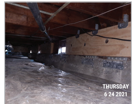
POST-RETROFIT CRAWL SPACE 2
