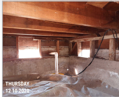
PRE-RETROFIT CRAWL SPACE 1
