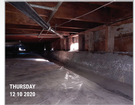
PRE-RETROFIT CRAWL SPACE 2
