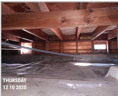
PRE-RETROFIT CRAWL SPACE 3
