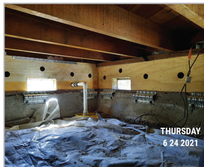
POST-RETROFIT CRAWL SPACE 1
