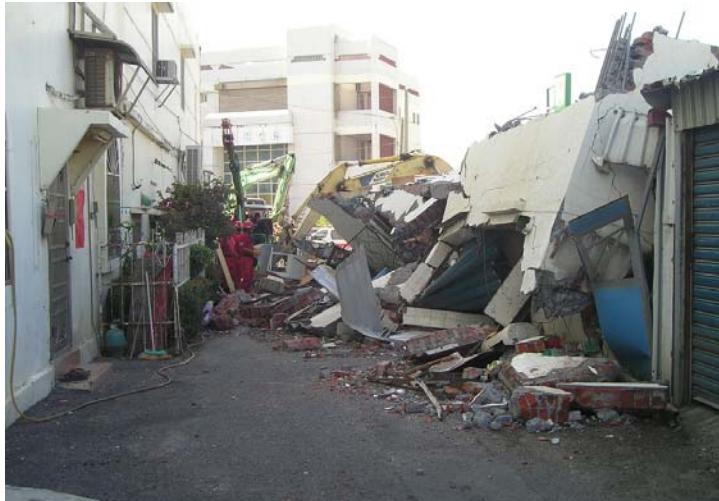
Fig. 8 Back view of the collapsed furniture store
