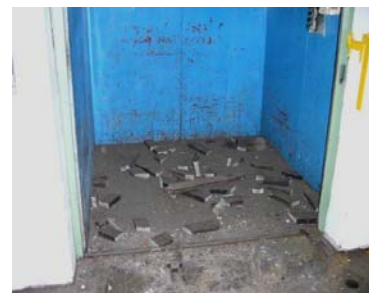
Fig. 18 CW iron plank fell in passenger cart
