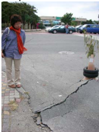
Fig. 19 Heave of pavement near Nanwan
