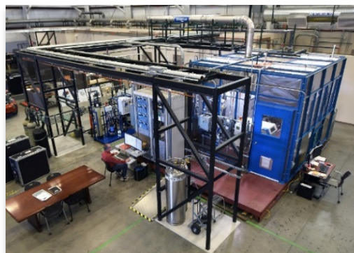
Figure VHTR 8. 25 kW HTSE Test Facility in DETAIL within the INL Energy Systems Laboratory
