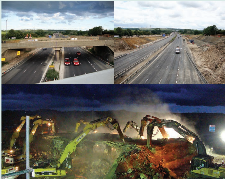
Top left and right: Saturday night and Sunday morning on the M1. Bottom: teams working for the Highways Agency attack the structure overnight
