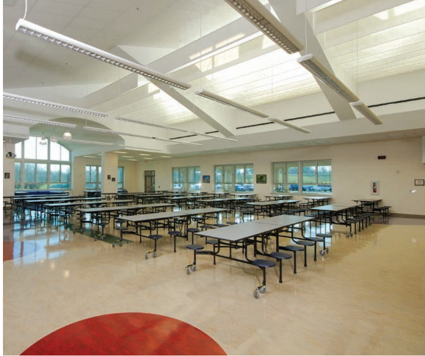
Ceiling baffles (top right) restrict the sunlight in the cafeteria and other south-facing rooms.
