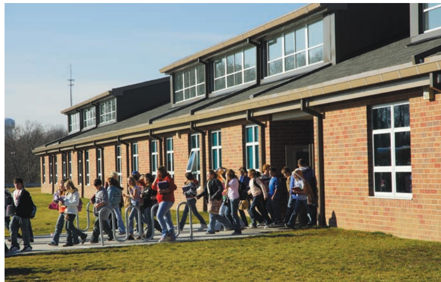
The roof dormer glazing provides natural light to classrooms. After daylighting was successfully implemented at Twenhofel, the Kentucky Department of Education reduced the artificial lighting requirements for daylit classrooms to 40 footcandles.
