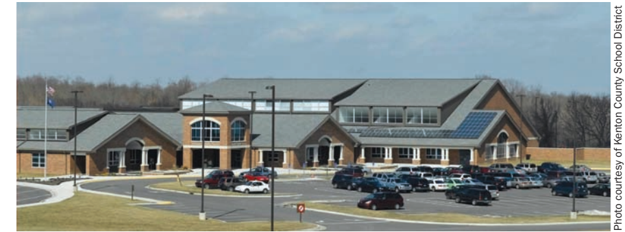
A rainwater harvesting system stores storm water runoff in a 100,000 gallon underground tank. This water is used to irrigate the athletic field and serves the water requirements of toilets and urinals in the school.
