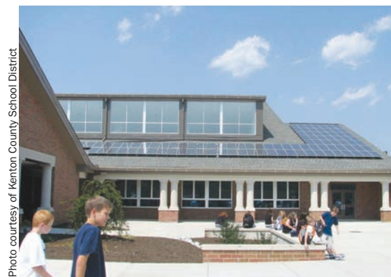
The 22 kW solar photovoltaic array, seen from the front entrance of the school, consists of 26 crystalline silicon PV panels, each rated for 110 watts and configured in four arrays that are each connected to a 6,000 watt dc/ac power inverter.
