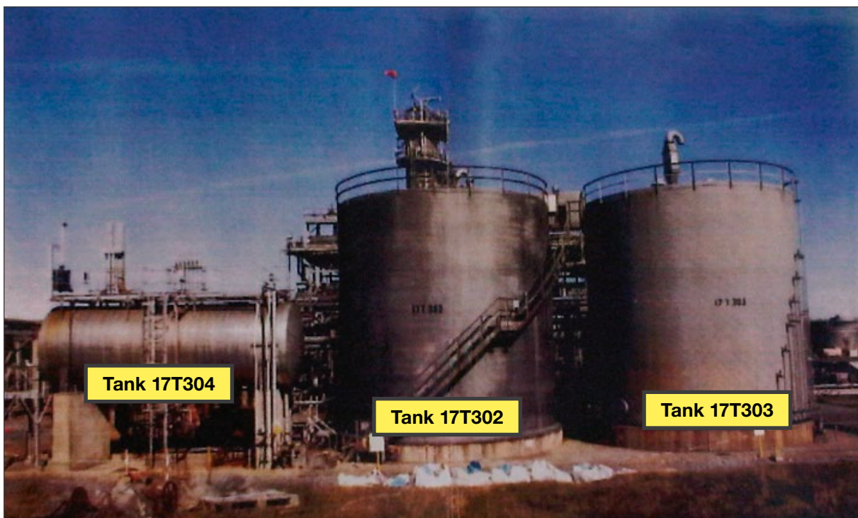
Figure 2 Pre-incident photograph of ARU tanks
