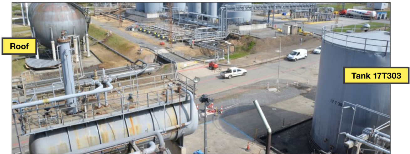
Figure 13 Post-incident photograph of tank roof location
