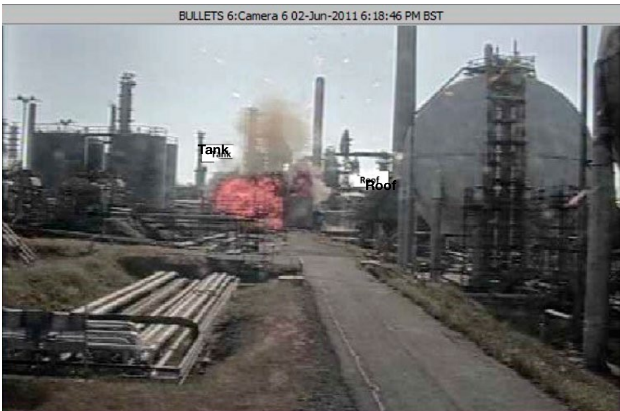
Figure 12 CCTV image showing ejection of tank 17T302 roof
