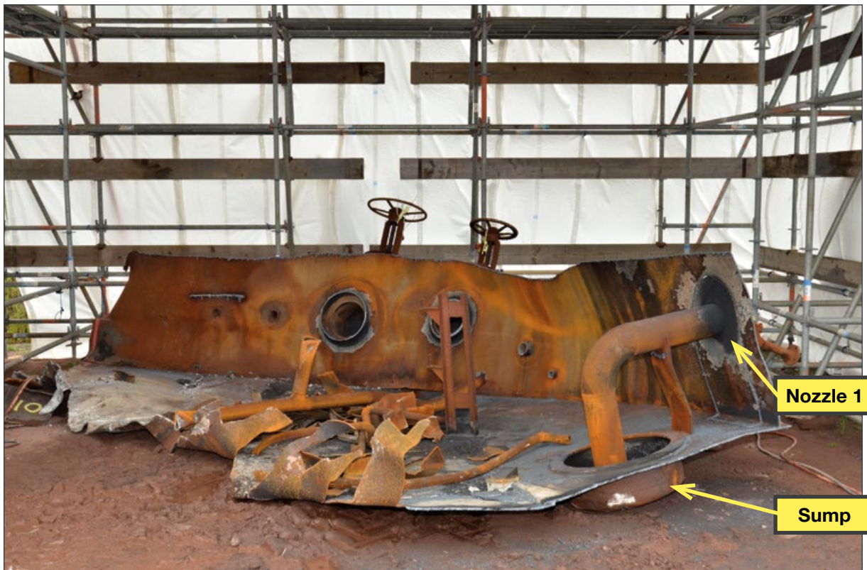
Figure 5 Post-incident section of tank 17T302 showing drain equipment
