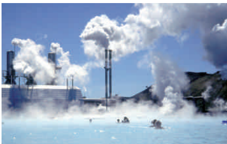
The 75MWe generating plant by the Blue Lagoon that also provides heat for a large district heating scheme.
