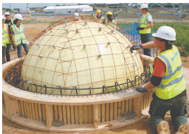
'Nuclear power station' dome ready for the concrete
