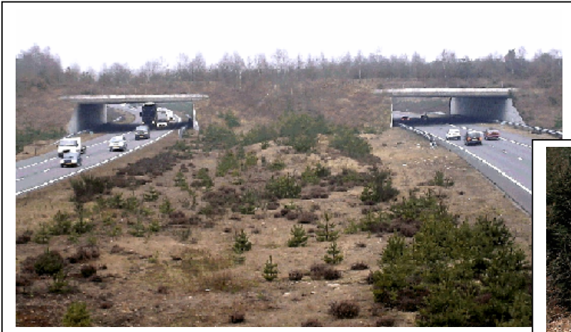
Figure 7 - Ecoduct over A1. When it was implemented, the road was already constructed and in operation. There is also a noise barrier, which consists in an embankment of soil and vegetation.
