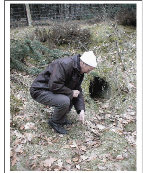
Figure 9 - Badger tunnel, installed on an existing road. The tracks on the ground show that it has been used frequently by badgers.
