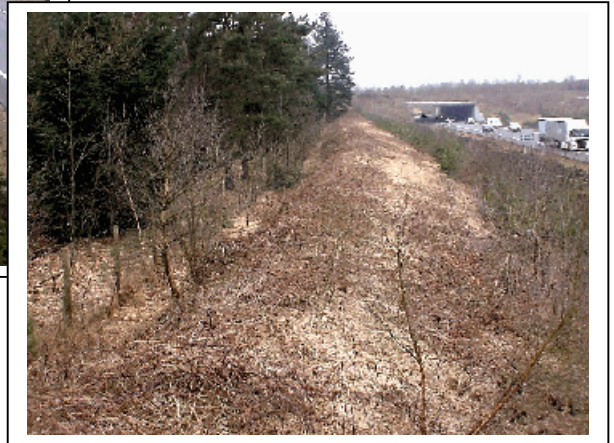
Figure 7 - Ecoduct over A1. When it was implemented, the road was already constructed and in operation. There is also a noise barrier, which consists in an embankment of soil and vegetation.
