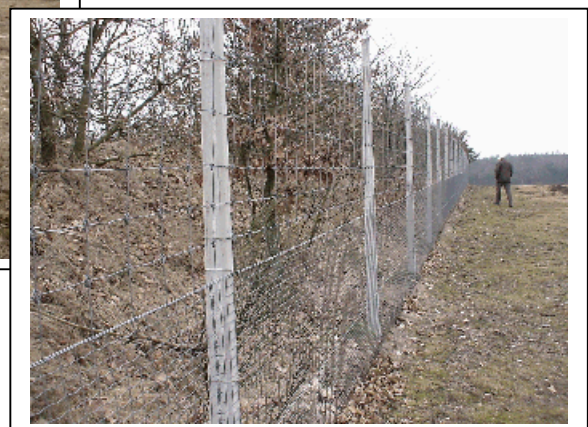
Figure 10 - Ecoduct over a highway. On the right is visible the combined fence: to large game above and amphibians below.
