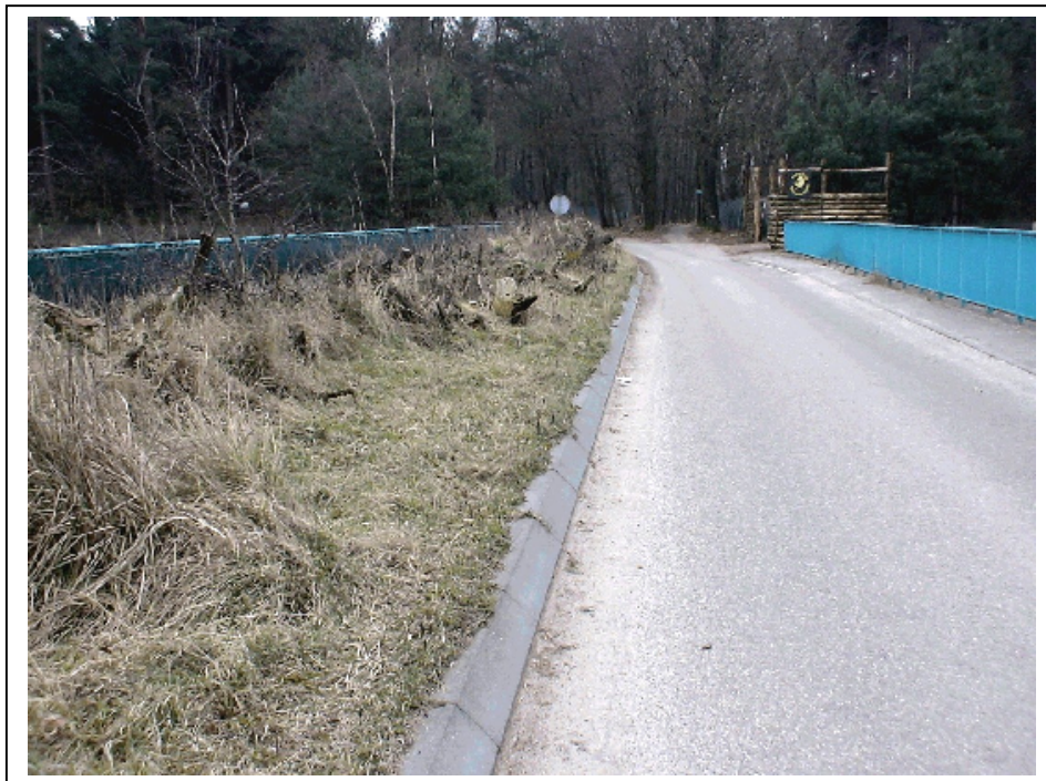
Figure 6 - Viaduct over A28. It were made some adaptations in order to be used by fauna: wall of tree-stumps and net to hide the cars.
