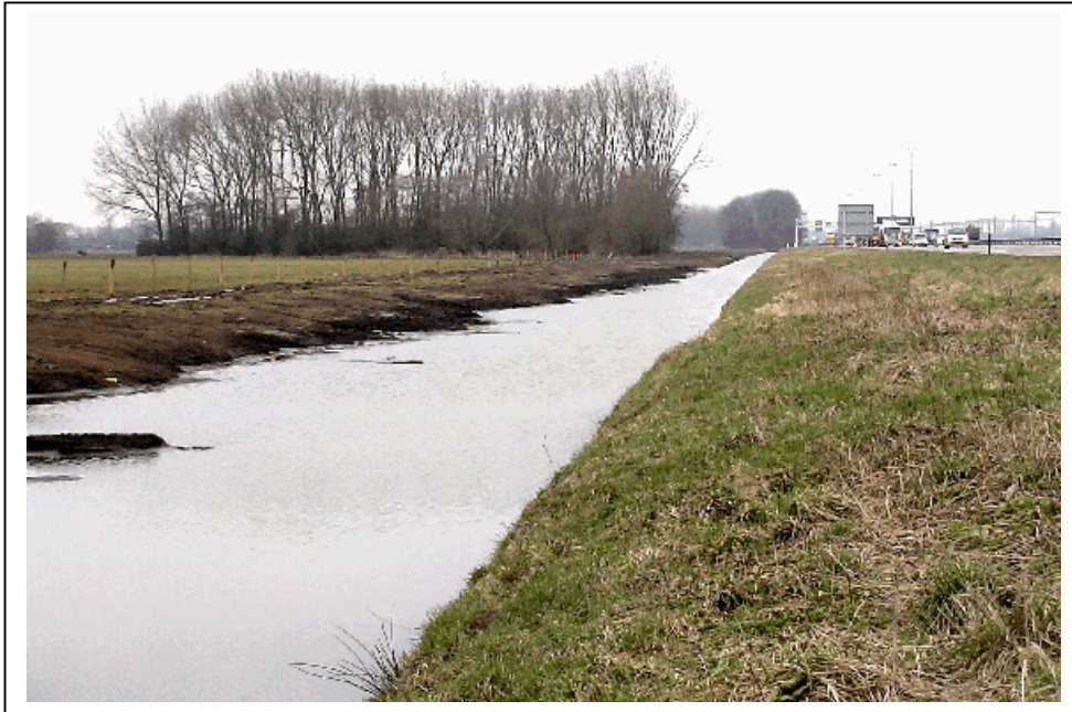
Figure 4 - The waterside of this ditch along the highway is being reconstructed in order to become less steep. This has the double effect of preventing animals from drowning and promoting more flora diversity and abundance.
