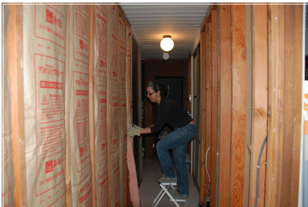
A woman installs insulation in her home. Photo: Nick Nguyen
