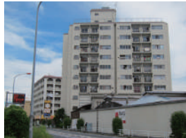
<Outer appearance before construction>
