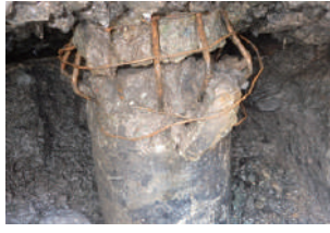
<Damaged pilings>
