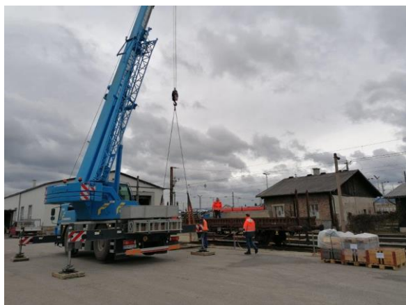
Construction of fuelling station
