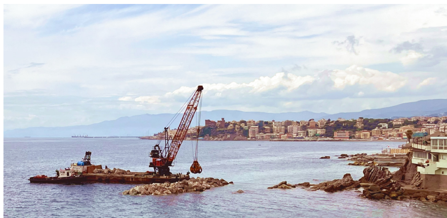
Figure 5. A pontoon adding new boulders to an already existing artificial reef at Quarto. The outer port of Genoa is visible in the background.
