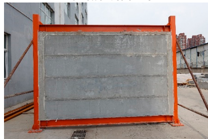
(f) The mould was removed after the concrete cures
