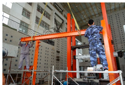
(a) The beam and brackets were connected
