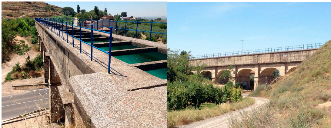
Figure 1. Coll de Foix Aqueduct located in Km 67 of CAyC.
