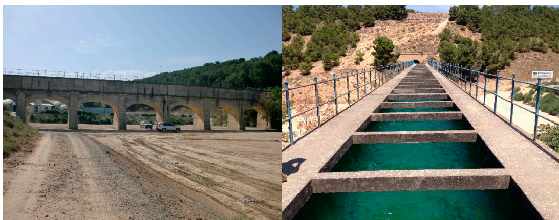
Figure 2. Capdevila Aqueduct located in Km 71 of CAyC.
