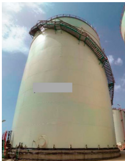
Figure 1. Exterior view of the vertical storage tank studied in this work.
