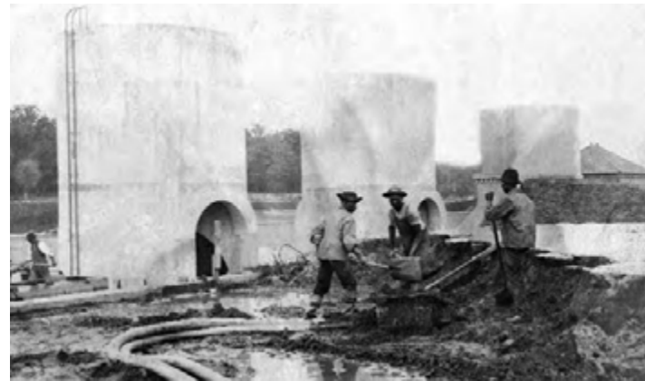
McMillan Sand Filtration Plant under construction (USACE photo)
