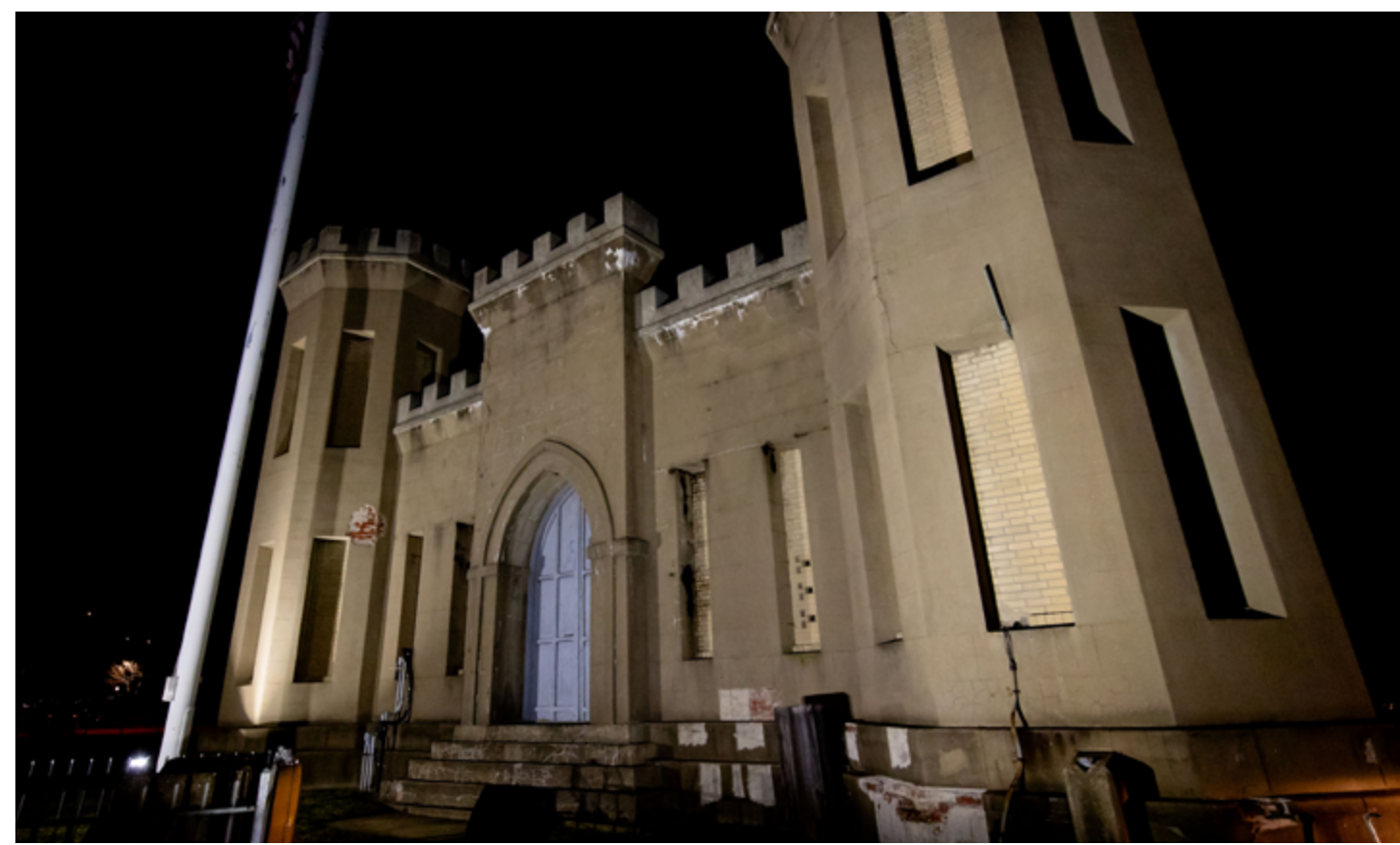
The Castle Gatehouse at the Georgetown Reservoir. (U.S. Army photo by Christopher Fincham)
