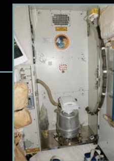
Waste Hygiene Compartment (WHC) collects urine and waste for processing.
