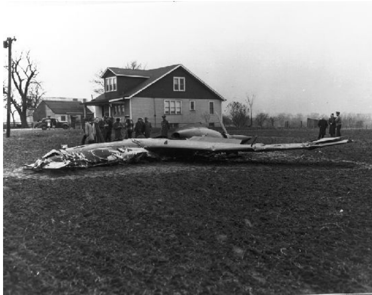
Figure 3.14: First XP – 55 crashed during stall characteristics test flight, 1943.
