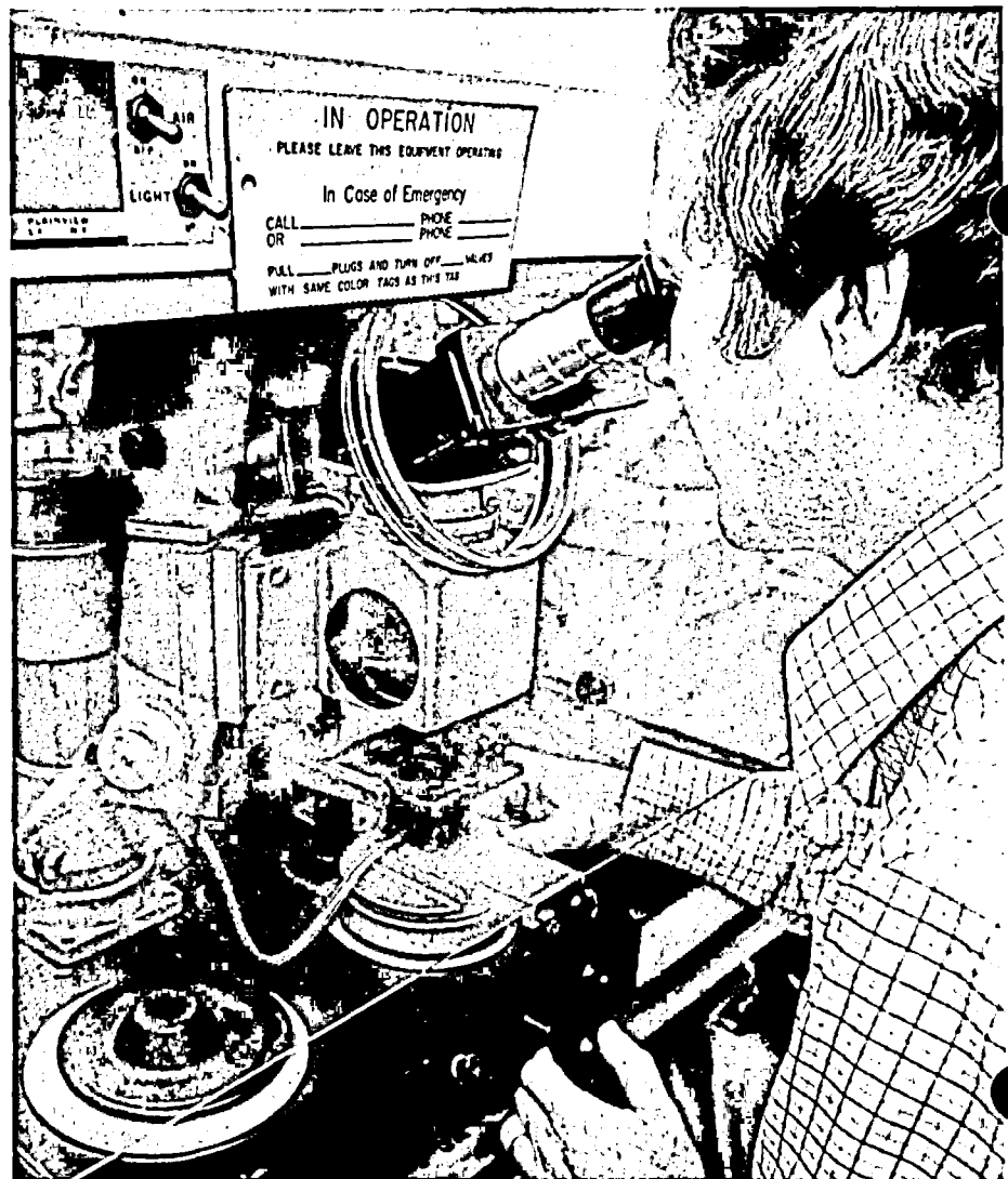
Photolithography processes are used for fabricating semiconductor components.
