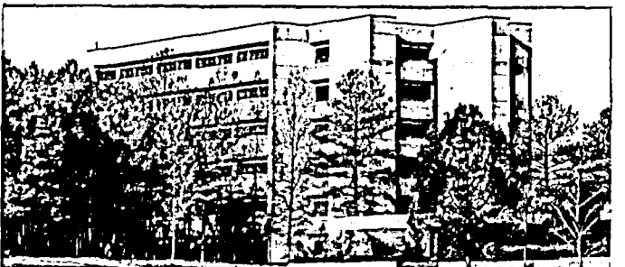
George Watts Hill Building
