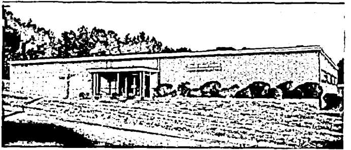
Energy and Environmental Research Annex
