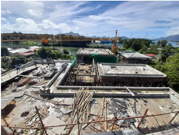
Major concrete works have been completed
