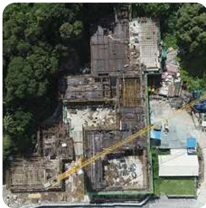
Aerial view of SBC House under construction
