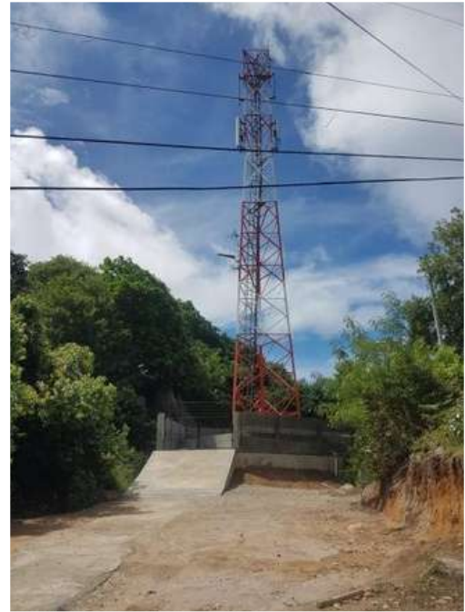
The new transmission tower at Fairyland
