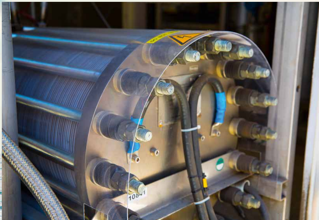
Figure 1: PEM electrolyzer
