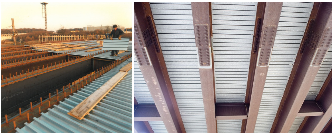
Fig. 2.25: Erection and bolted connections of the OAT5 Howald bridge in Luxembourg
