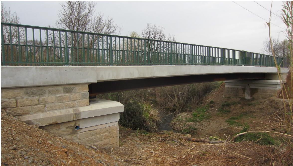
Fig. 2.6: Composite bridge after opening and some weeks of outdoor exposure, San Martin à Fontes, France
