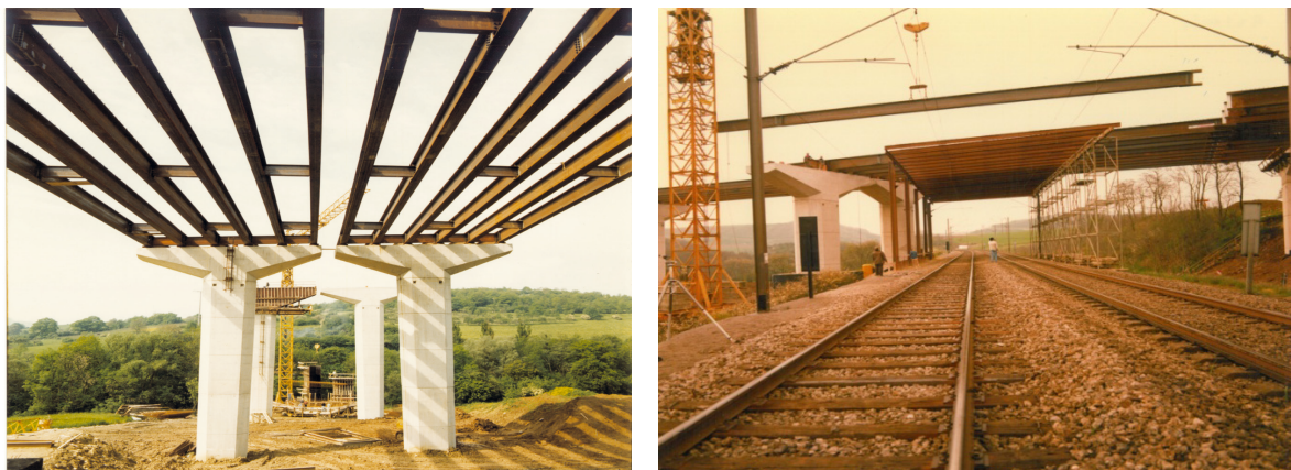
Fig. 2.14: Syre viaduct erection phase, A1 motorway in Luxembourg
