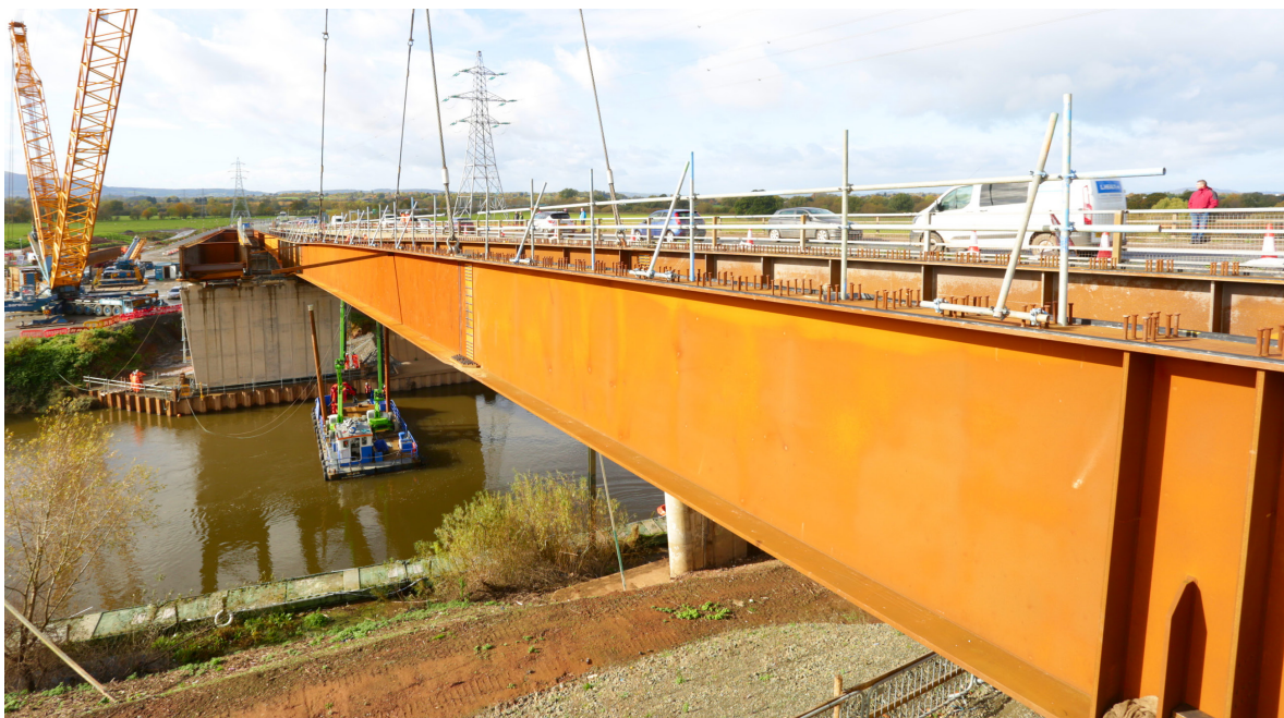
Fig. 2.32: Erection of the Carrington Bridge in Worcester, England
