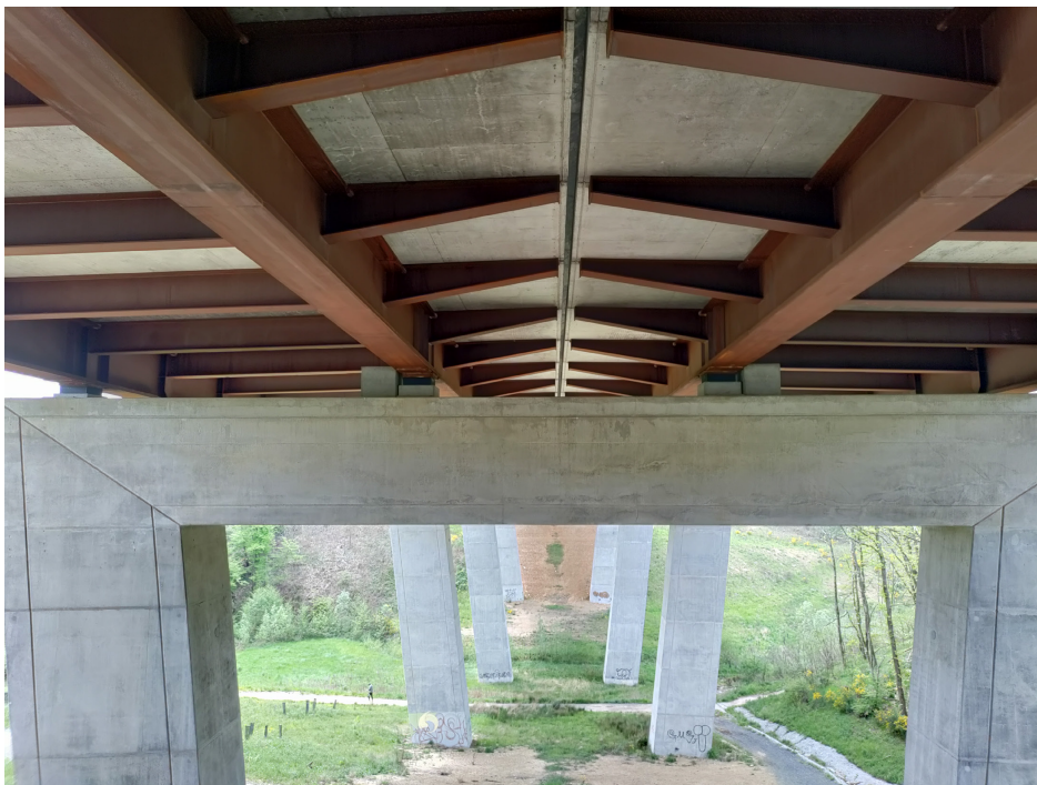
Fig. 2.18: Viaduc de Sémanet in Dardilly (Auvergne-Rhône-Alpes, France) built until 2018
