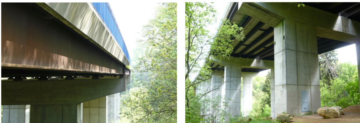
Fig. 2.12: Mamer viaduct, A6 motorway in Luxembourg
