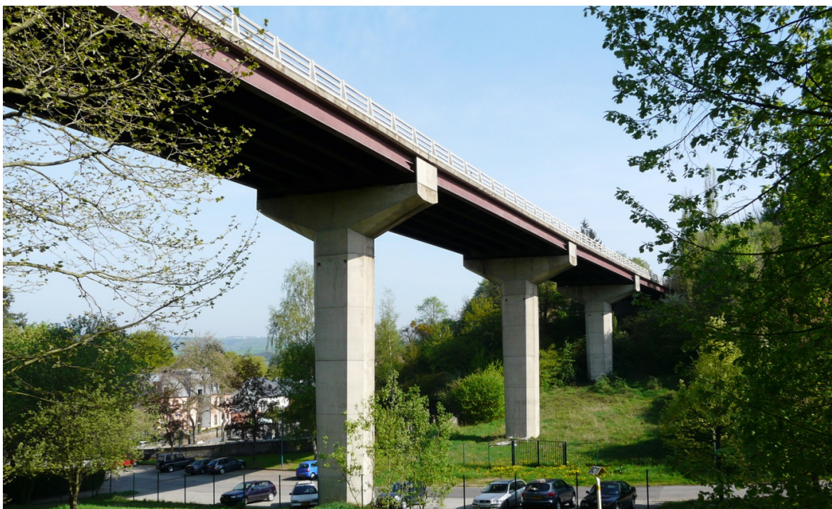
Fig. 2.10: Ditgesbaach viaduct, access to A7 motorway in Luxembourg
