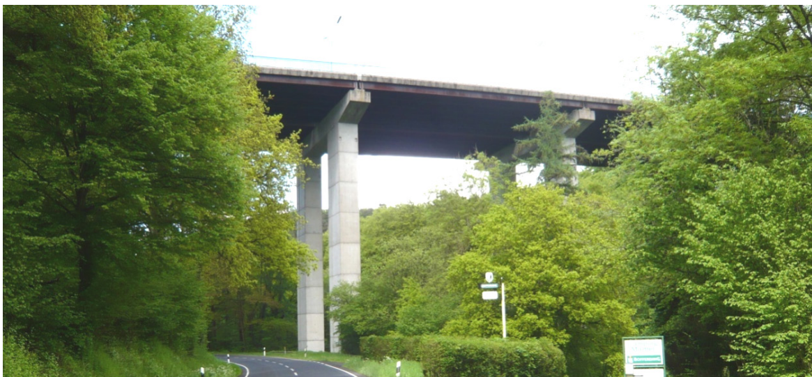
Fig. 2.11: Mamer viaduct, A6 motorway in Luxembourg
