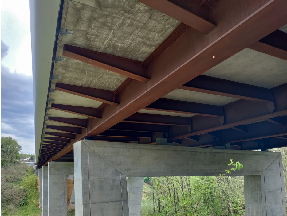
Fig. 2.17: Viaduc de Sémanet in Dardilly (Auvergne-Rhône-Alpes, France) built until 2018
