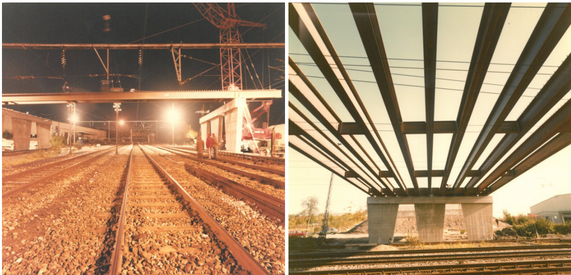
Fig. 2.24: Erection of the OAT5 Howald bridge in Luxembourg
