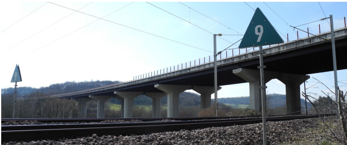
Fig. 2.13: Syre viaduct, A1 motorway in Luxembourg
