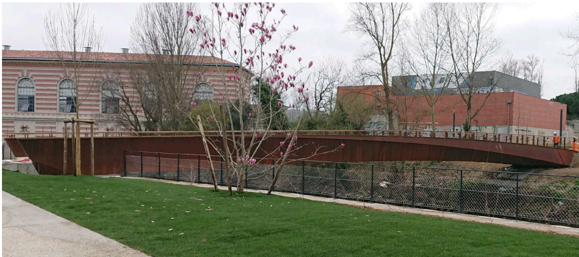
Fig. 2.33: Pedestrian and cycling bridge in Banleve, Toulouse, France
