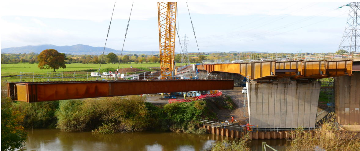
Fig. 2.31: Erection of the Carrington Bridge in Worcester, England
