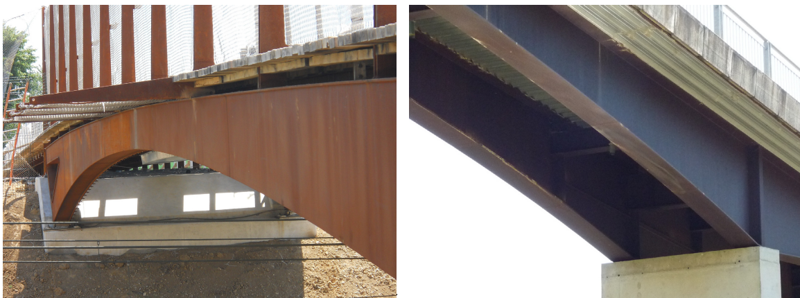
Fig. 5.1: Example for a very young oxide layer while erection (left) and a fully formed oxide layer after many years in service (right)
