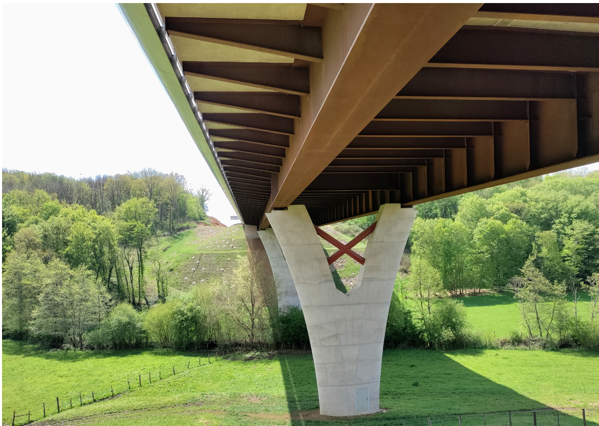
Fig. 2.7: Viaduc de la Scyotte in Grattery, France, completed in 2018
