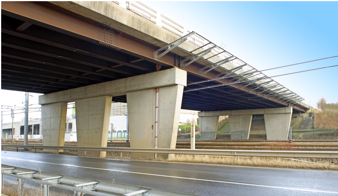
Fig. 2.23: OAT5 Howald bridge over railway line and roadways in Luxembourg
