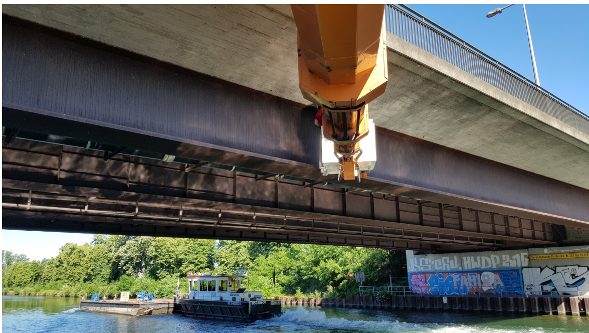
Fig. 2.16: Composite Bridge over a canal in Herne, Germany (construction year: 1975, photo: 2019)
